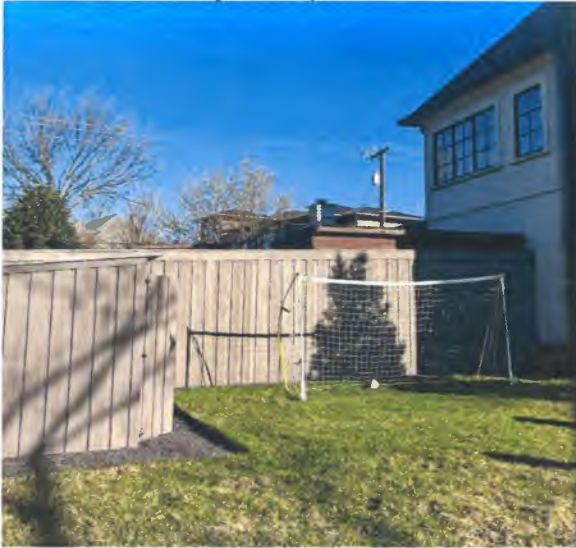
4. 6143 Royalton (structure built in side yard; possibly after CO)
