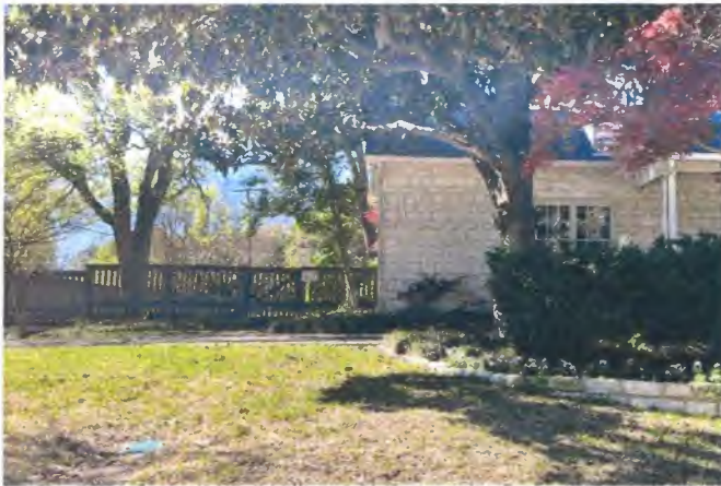
13. 11110 Lawnhaven (structure in side yard behind fence, prob built after CO)
