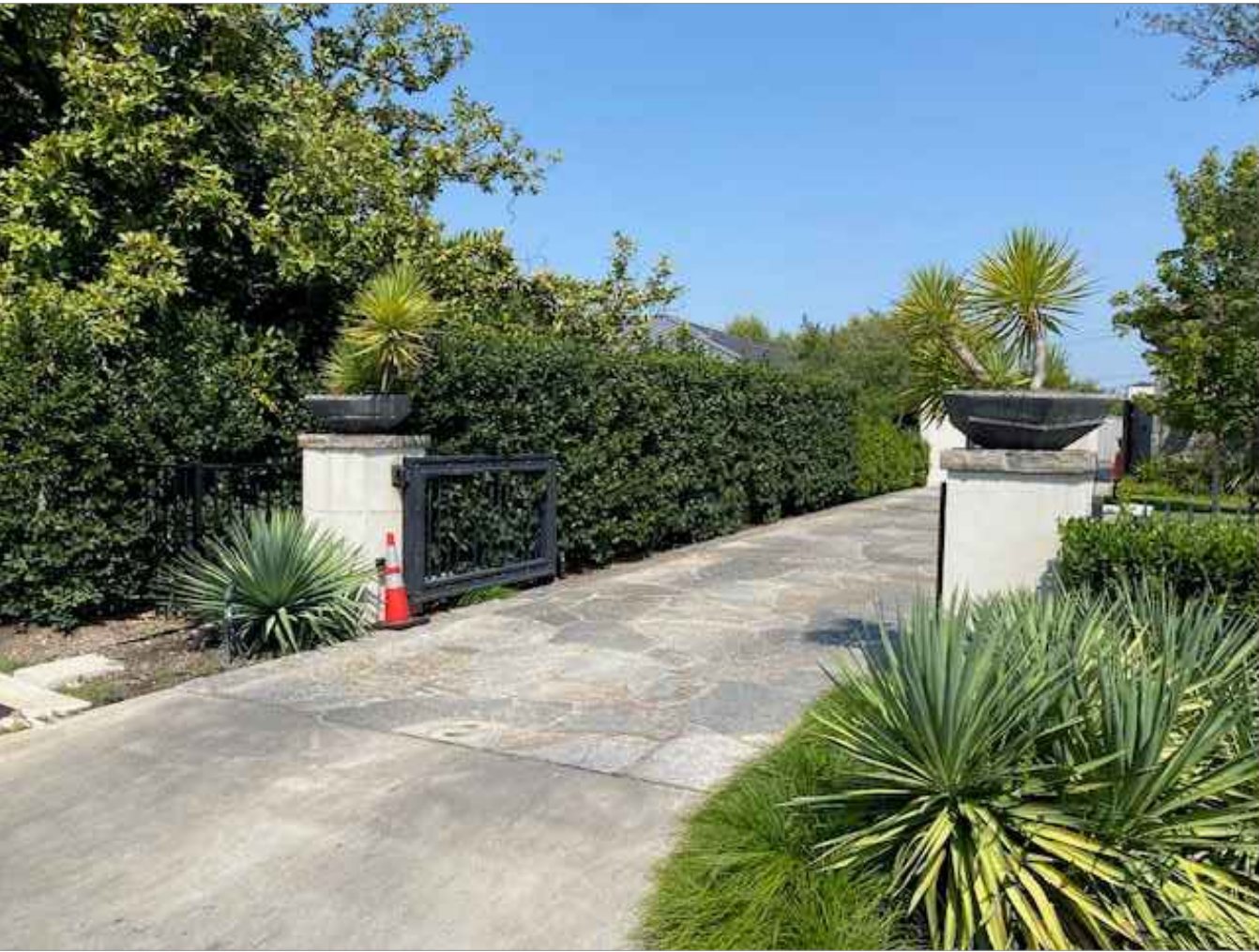
EXISTING WEST SIDE PROPERTY LINE
