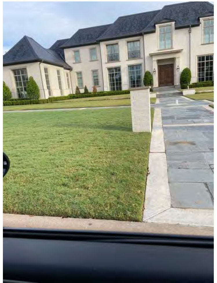
4651 Catina The front yard faces the house asking for an adjustment Notice the open front yard
