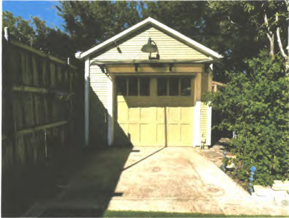
EXISTING 1-CAR GARAGE – 205 S Windomere – East front elevation
