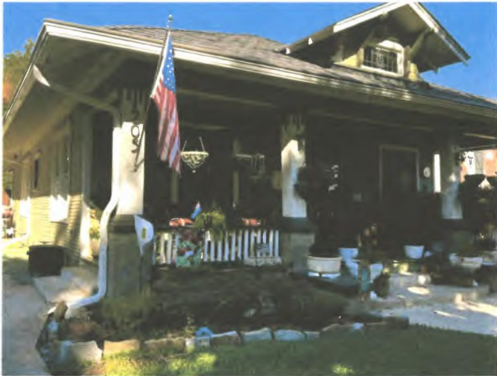
EXISTING MAIN RESIDENCE – 205 S Windomere – front porch columns & dormer detail
