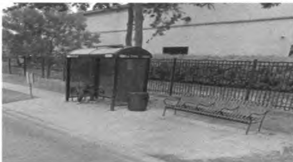
Figure 3 North Bus stop location on S Malcolm X Blvd, just north of the project site
