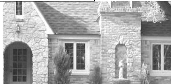
Stained glass / corbelled chimney with niche
