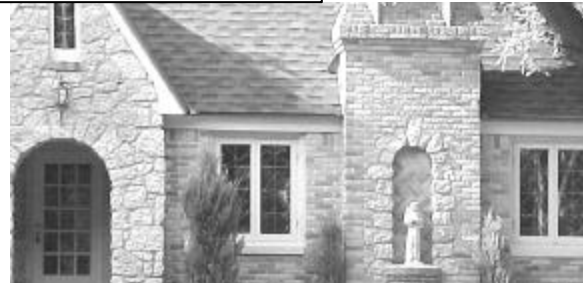
Stained glass / corbelled chimney with niche
