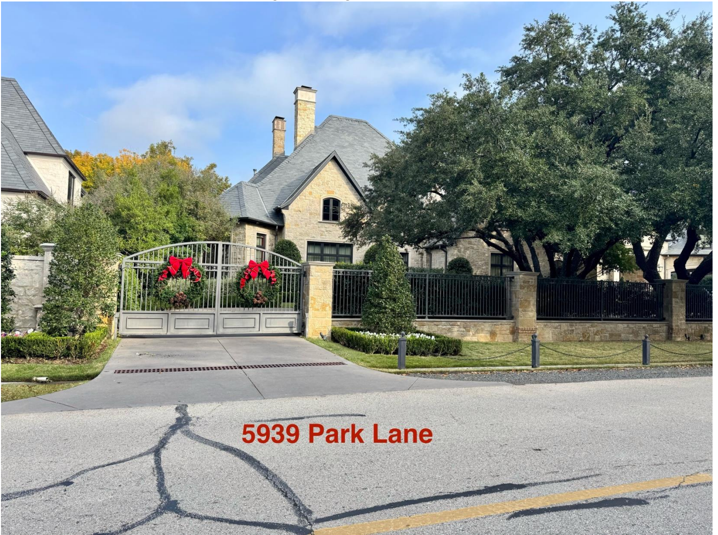
6. 5939 Park Lane – Pillars are more than 8' high from the ground
