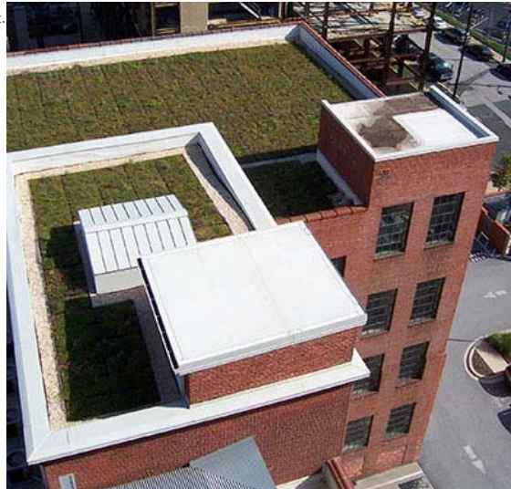
Figure 22. Installation of both cool and green roofs in an urban environment.
