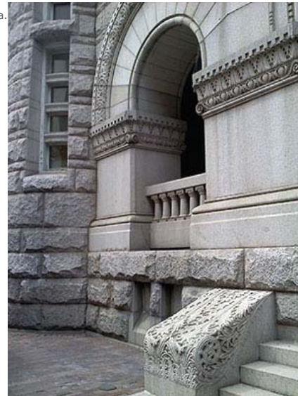
Figure 3. Stone walls with substantial mass have high thermal inertia.
