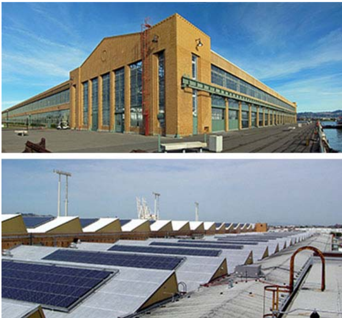
Figure 23. Solar collectors installed in a compatible manner on low sloping sawtooth monitors. Top Photo: Neil Mishalov, Berkeley, CA.
