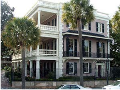
Figure 5. The side porches of this house in Charleston, SC, shade the large windows and provide outdoor living spaces that take advantage of sea breezes.
