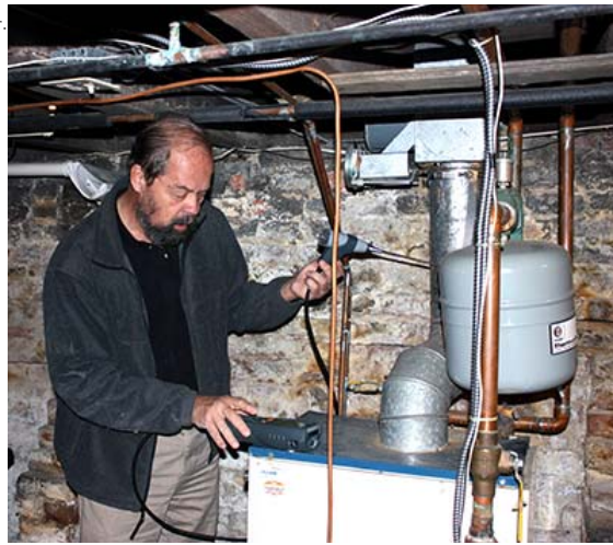
Figure 9. An energy auditor tests the efficiency of a boiler.
