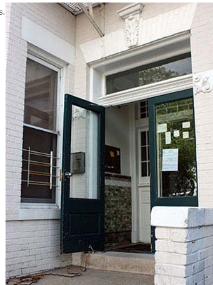
Figure 16. Historic vestibules retain conditioned air in the living spaces.
