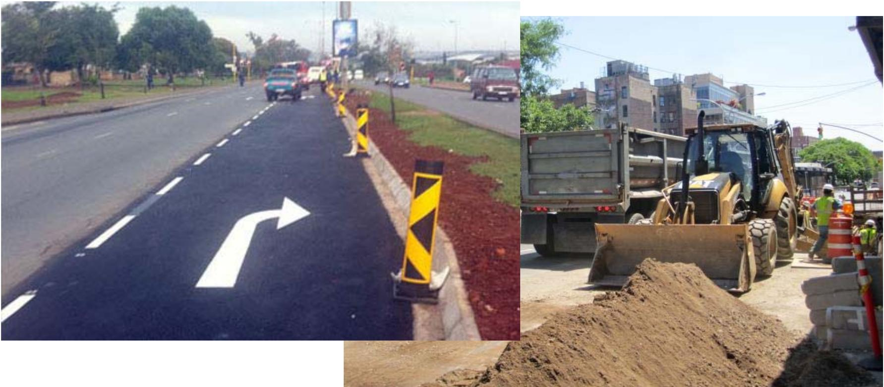
Street and alley repairs by the Dallas Water Utilities are associated with pipeline replacement. For asphalt streets the City policy requires that an entire lane be reconstructed at the location for where the pipeline is replaced. From joint to joint for concrete streets.
