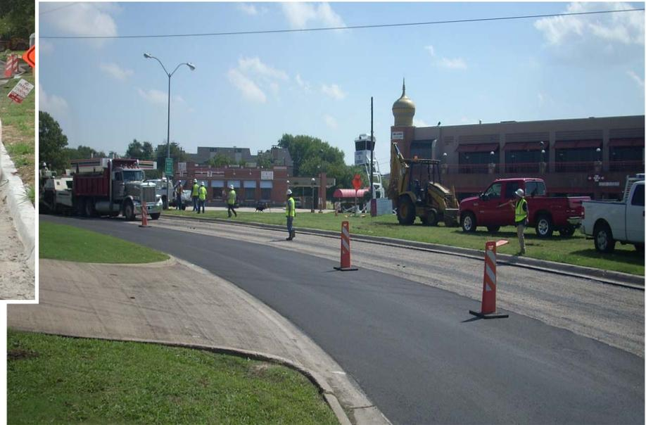
**Re-Surfacing** – This treatment removes the entire asphalt surface, and pulverizes and recycles the old material with new asphalt binder. The new asphalt surface is then placed over the entire surface, compacted, and smoothed to a proper finish. Curb and gutter repair, if needed, is accomplished with the re-surfacing efforts.
