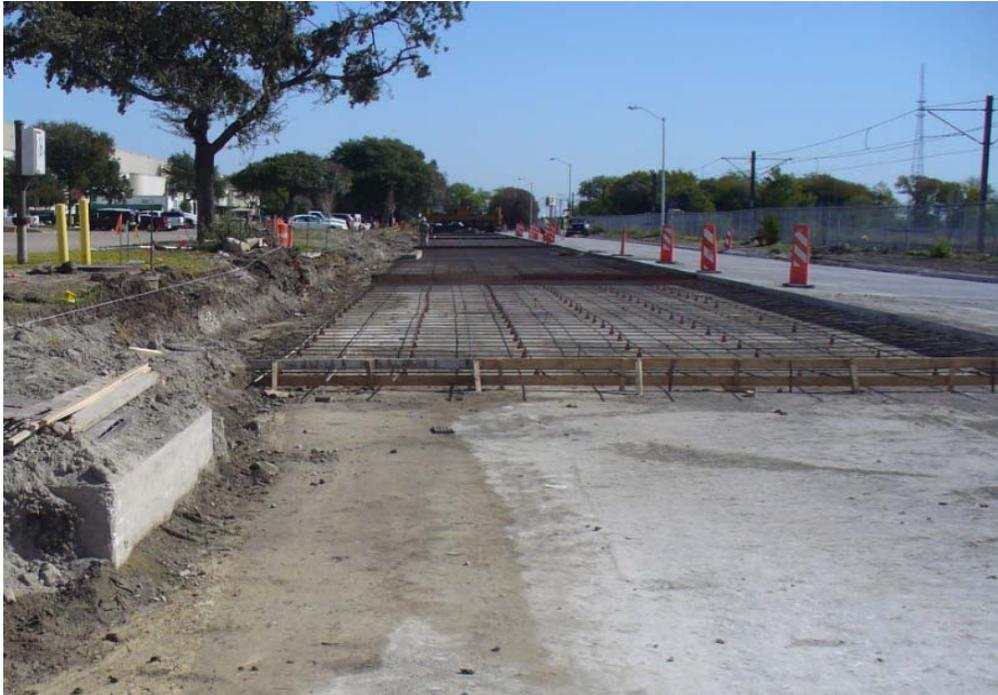
**Reconstruction** - This process is the removal of an existing street with extensive failures and/or badly deteriorated condition. In the process, the pavement is broken and removed (and often recycled), as is the base. Drainage concerns are addressed with this process. The sub-base may be reconditioned as needed, then a new base is placed and compacted. The new concrete surface pavement is then placed, as shown above. The construction work is outsourced under bond-issued funding.
