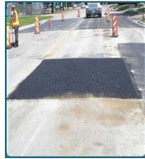
**Slurry Seal** - This treatment for CONCRETE STREETS WITH ASPHALT SURFACE consists of a ¼-inch layer of sand and fine stone mixed with asphalt emulsion. This seals and smooths the surface and conceals scars from previous repairs. It is used predominately for residential roads with curb and gutter. The work is outsourced to a specialized contractor – after Street Services performs preparation work (such as minor base repair and crack sealing).
