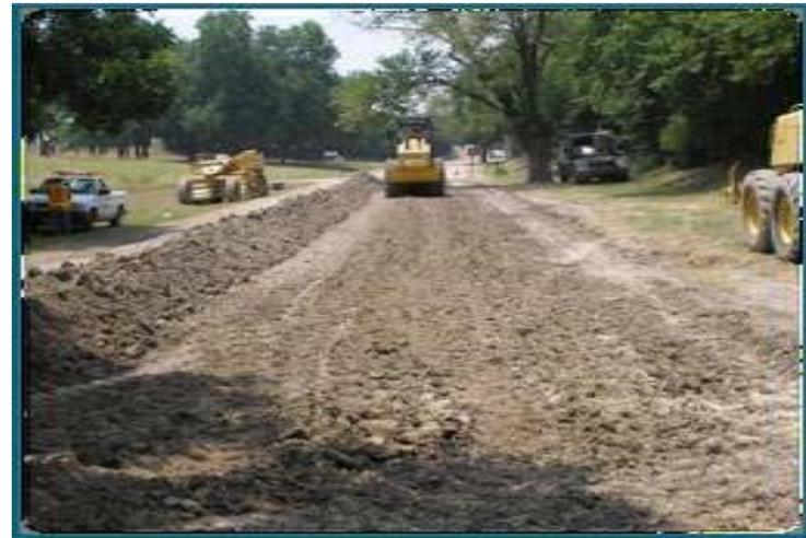
**Rehabilitation** - A treatment for ASPHALT STREETS when a large portion of the surface and the base have deteriorated to an unsatisfactory level. It includes the full-depth repair of base failures, followed by a chip seal, and a new two-inch layer of hot mix asphalt placed over the entire treated segment. Candidate streets are predominately residential asphalt surfaced streets without curb and gutter. **Cost:** \$160K per lane-mile. **Life:** 10-12 years.
