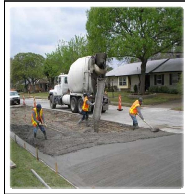
**Partial Reconstruction** - This is a method used on CONCRETE STREETS. It is **removal and replacement of large, failed sections**, including breakout and removal of old pavement, repair of any base failures, and placing new concrete. To be a candidate for this repair, residential and thoroughfare streets must have less than 25% of failed area.
