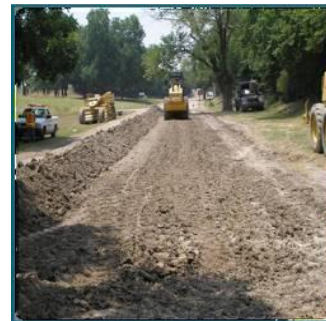
Asphalt Restoration for "E" rated streets
