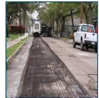
Asphalt Rehabilitation for "D" rated streets
