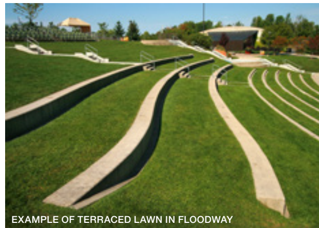
EXAMPLE OF TERRACED LAWN IN FLOODWAY
