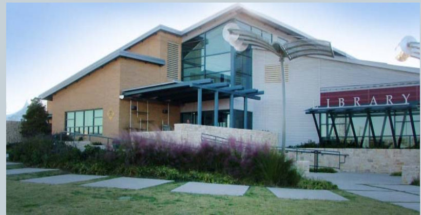
Timberglen Branch Library
