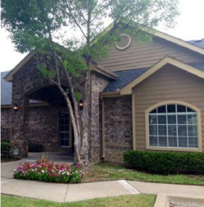
Park At Cliff Creek 280 Units CD 8
