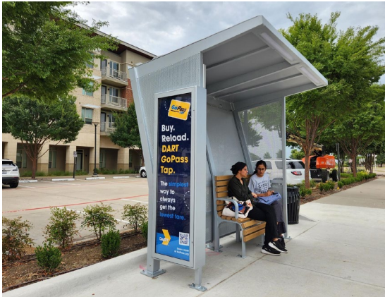
Modern Bus Shelters with Real Time Information
