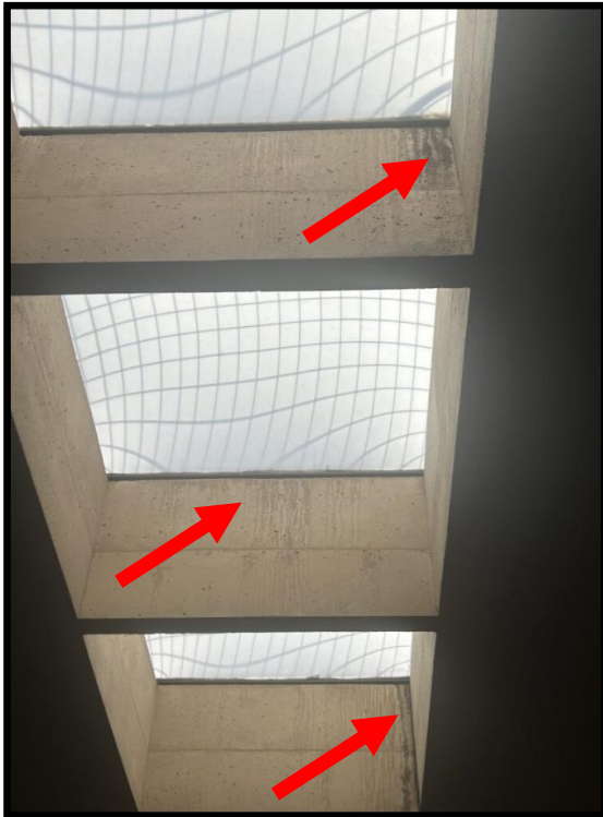
Stairwell roof skylight water infiltration
