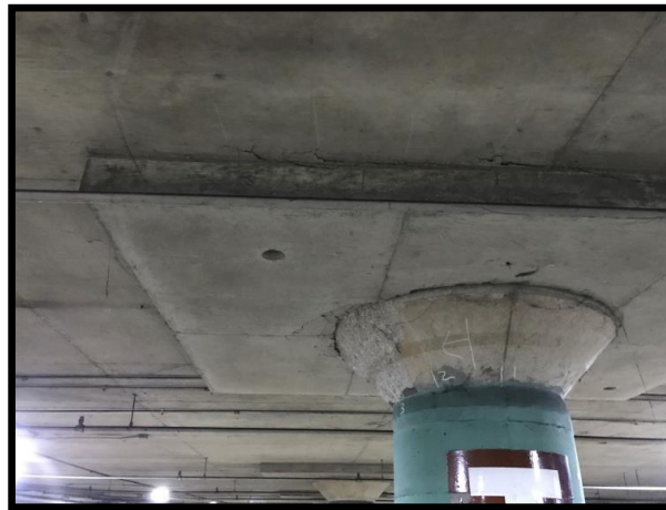
Structural failure: garage ceiling concrete spalling
