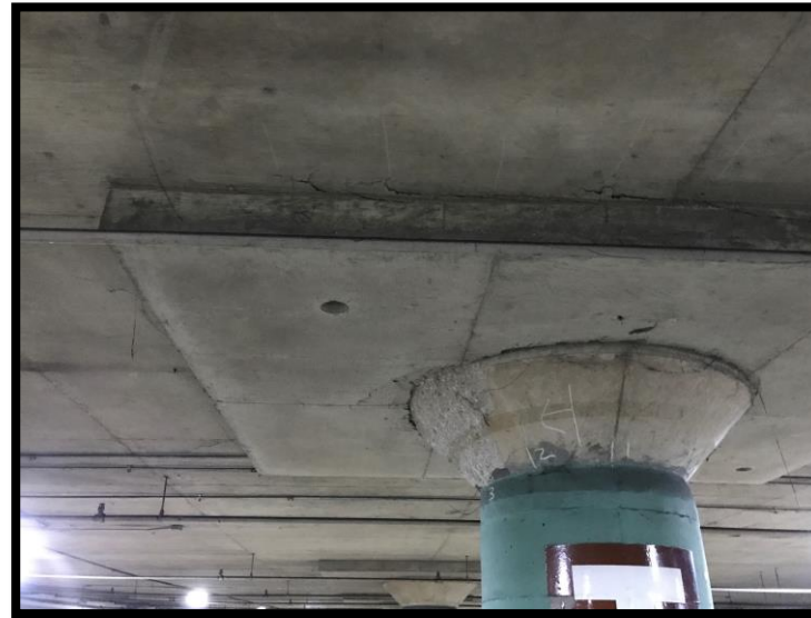
Structural failure: garage ceiling concrete spalling
