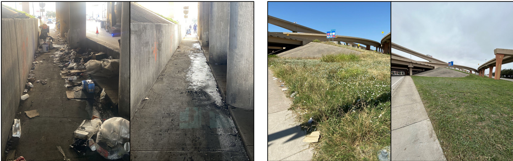
Maintenance provided along Walnut Hill and 635.
