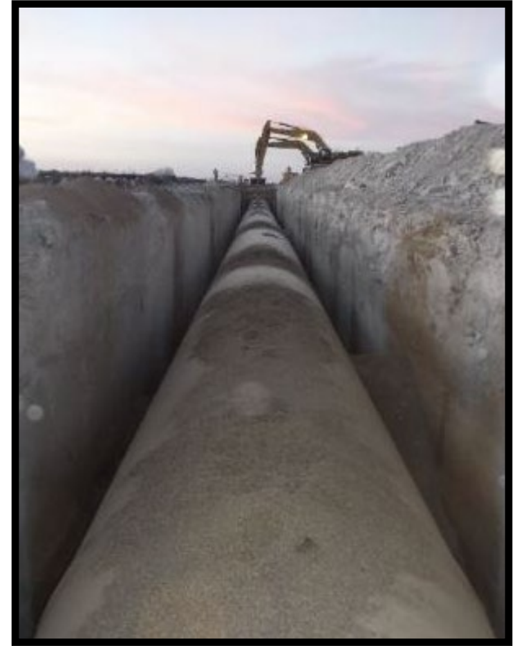
Installation of 108-inch pipe along IPL Section 17
