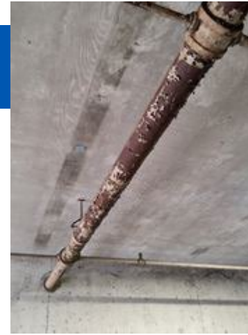
Corroded fire suppression piping indicative of aging sprinkler infrastructure in parking garage.
