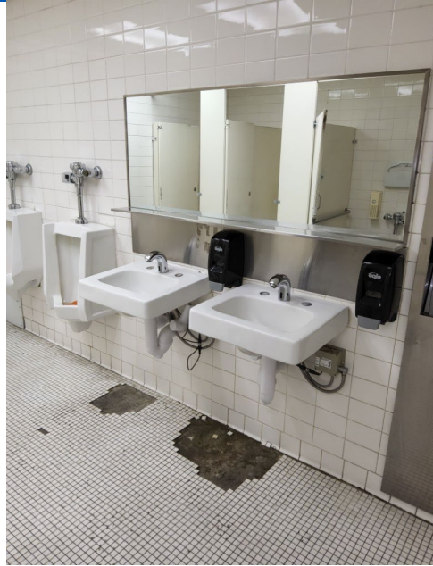
Deteriorated Finishes
