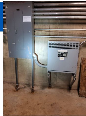
Aged electrical distribution equipment serving critical building and parking garage equipment.
