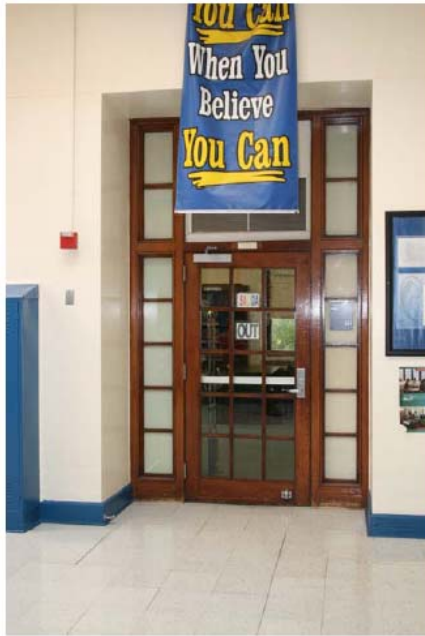
Typical original wood French doors, sidelights and transoms throughout building.
