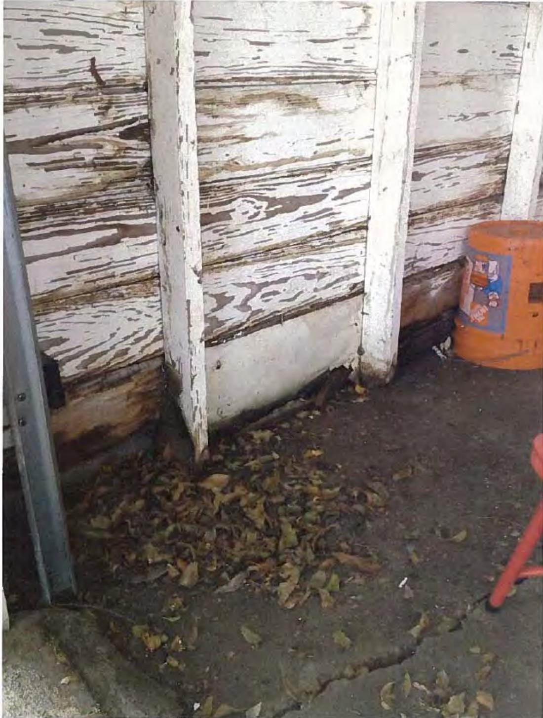
Picture of exterior wall with rotted framing and siding
