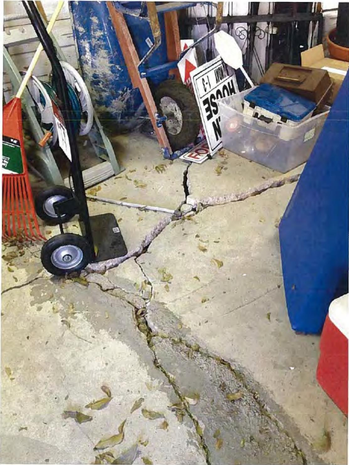
Interior concrete slab showing effects of foundation movement
