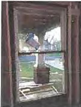
Window frame damaged not supported and warped. All hardware missing.
