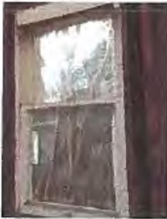
Window will not open, no counterbalance present. Hardware rusted shut. Frame warped.
