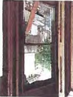
Frame bent and unusable, extensive damage to entire window.
