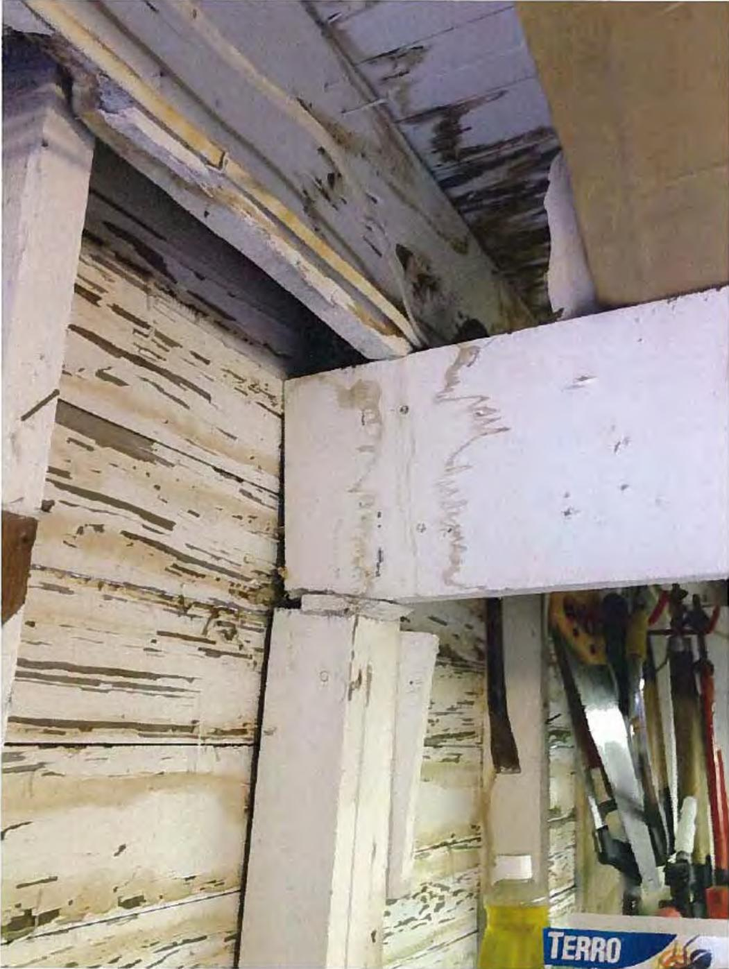
Beam connection built poorly and showing effects of structural movement
