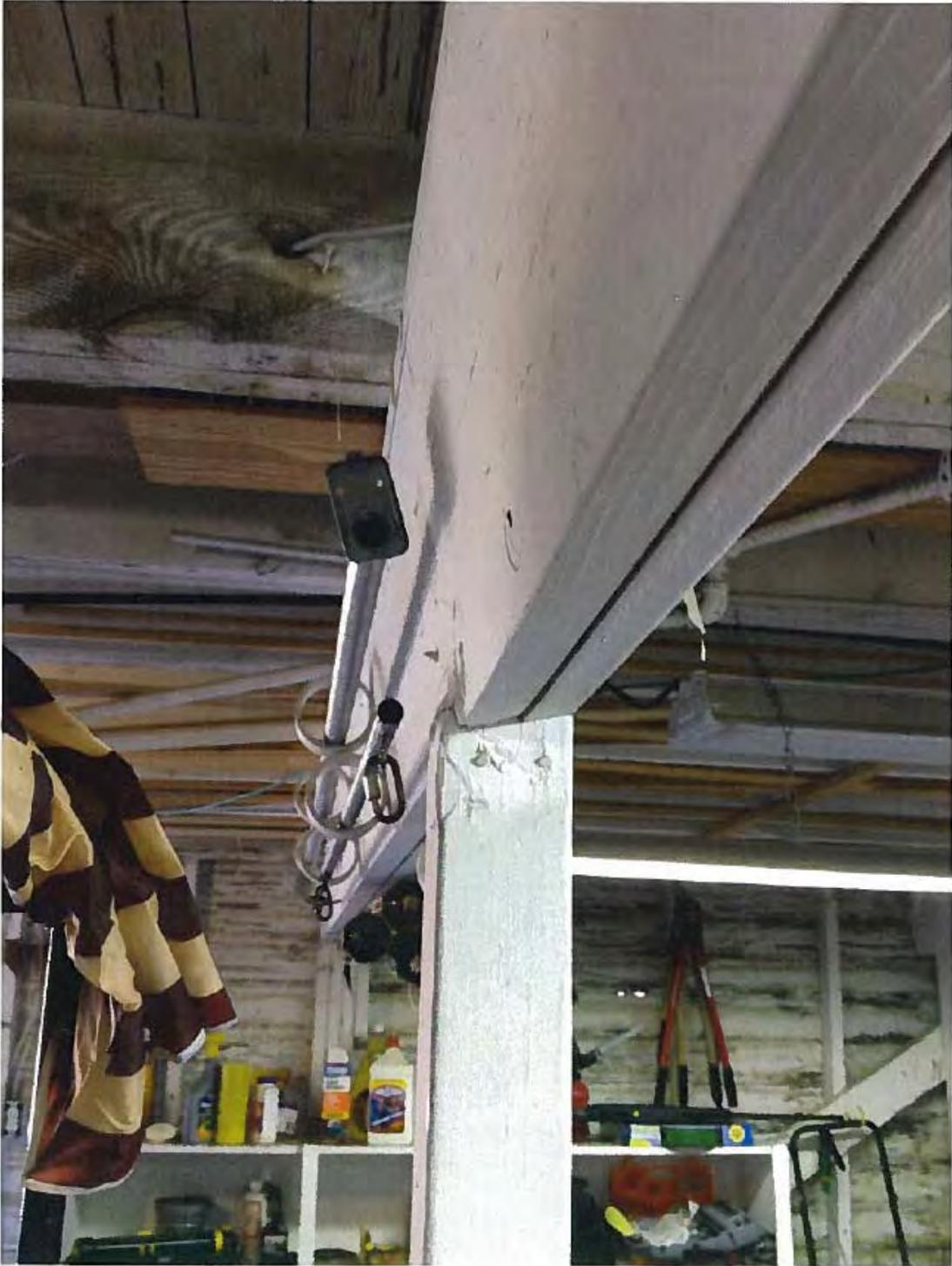
Interior beam connection built poorly and showing effects of movement
