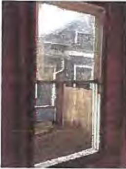
Window frame damaged not supported and warped. All hardware missing. Will not open.
