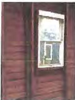
Window frame has warped, will not open and is painted shut. No counterbalance no support.
