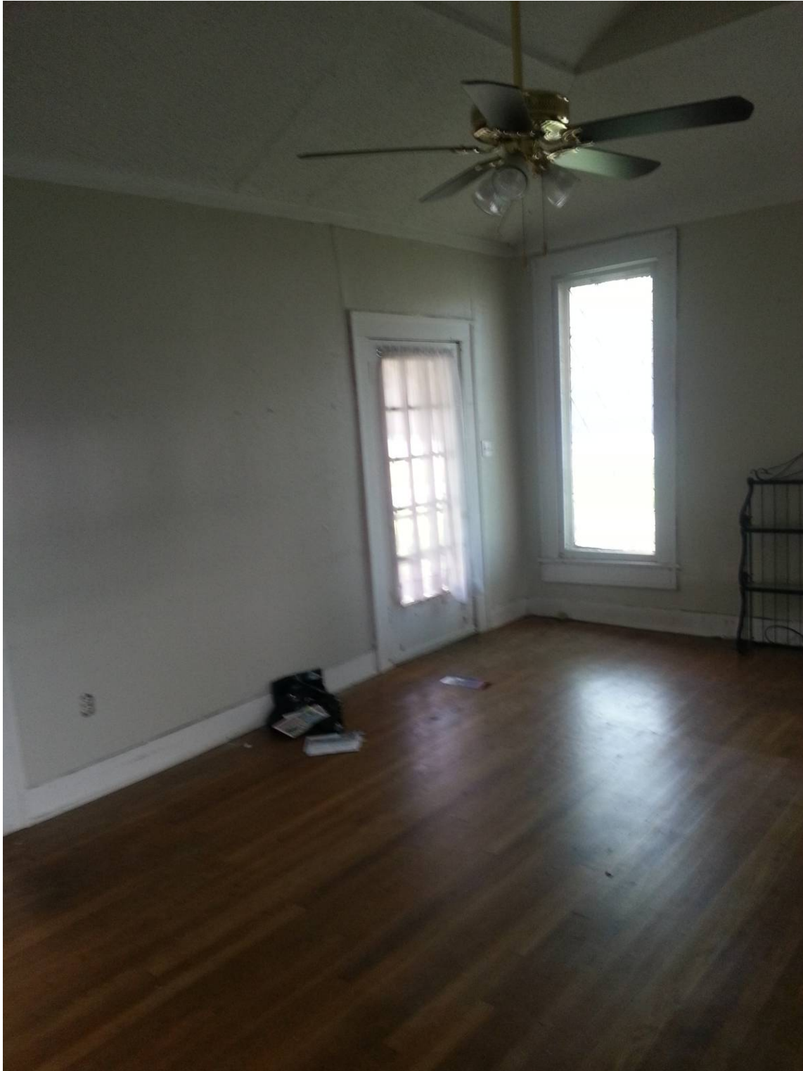
Existing front door is a 15-lite French door.
