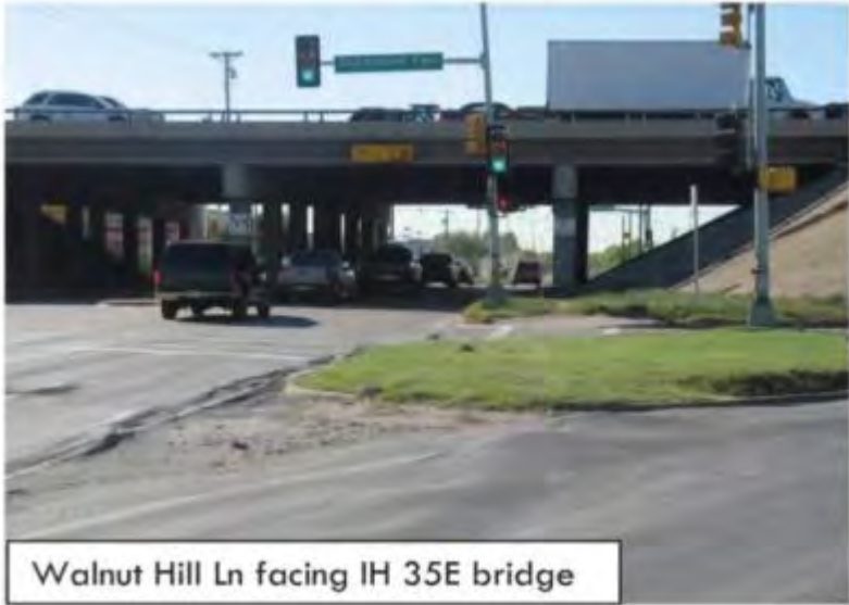
Walnut Hill Ln looking east
