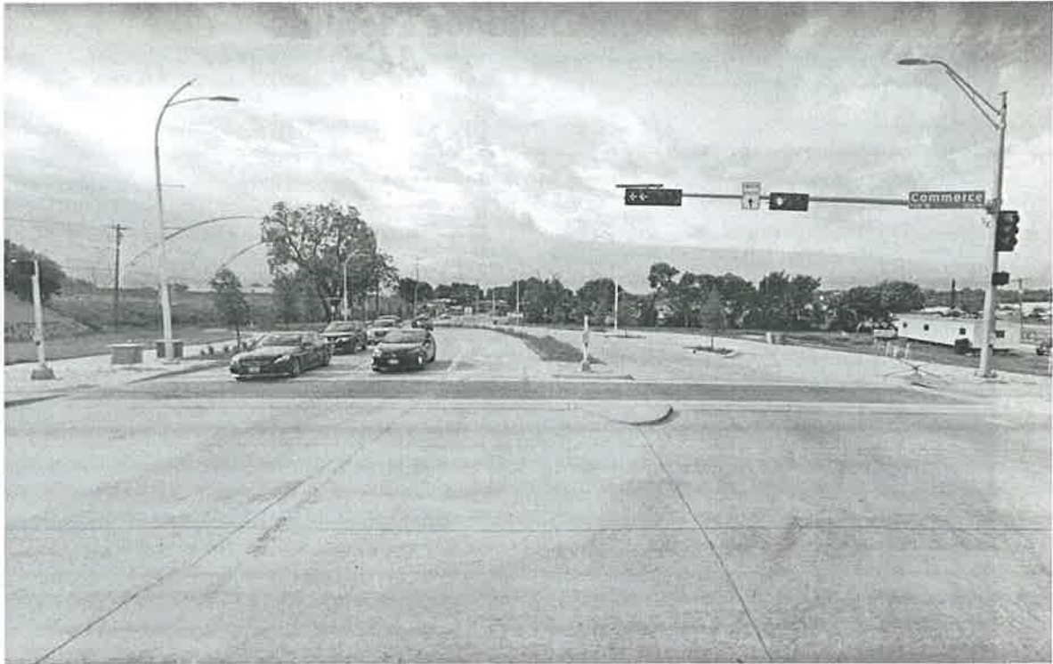
Figure 5 – Crosswalk across the southern leg of Beckley Avenue. Note the mid-street pedestrian push button.
