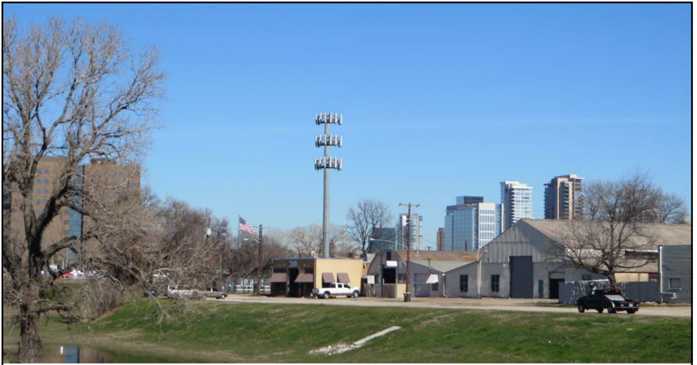
Extended 95' Monopole Tower
