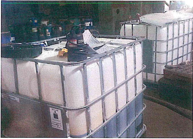
19. View of partially filled tote during chromic acid waste removal from sumps.
