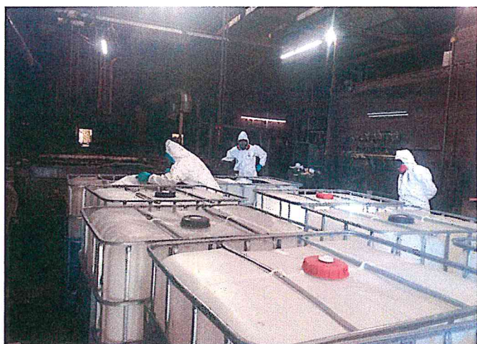
18. View of totes and SWS personnel during chromic acid waste removal activities.
