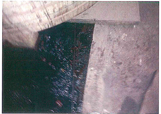
20. View of chromic acid waste in area of sump beneath poly tanks.
