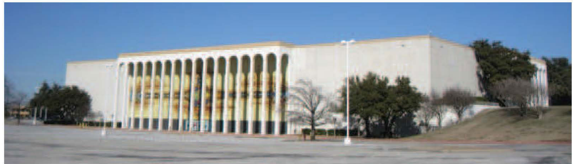
EXISTING CONDITIONS EXISTING MALL
