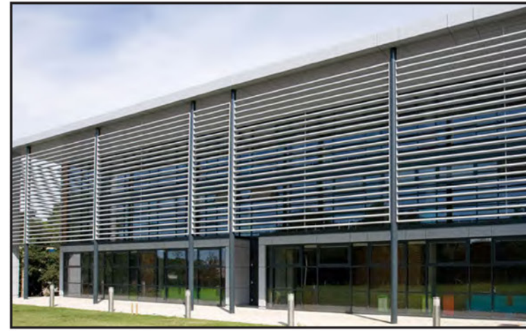
Painted Horizontal Metal Louvers, Canopies and Columns
