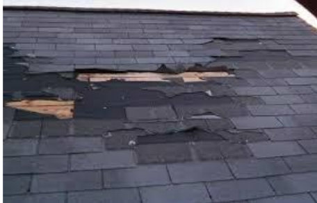
MISSING SHINGLES
