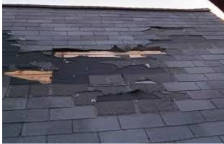
MISSING SHINGLES
