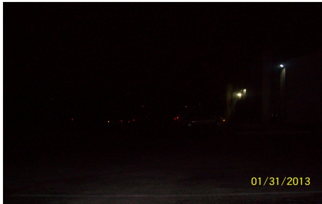
Violation - security light not in working order.
