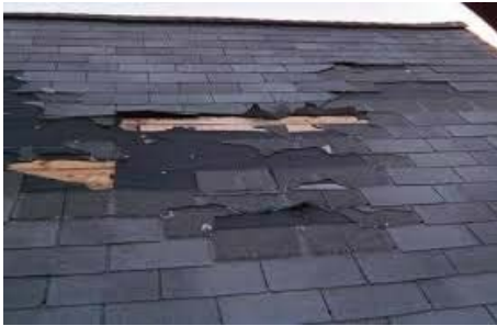
MISSING SHINGLES
