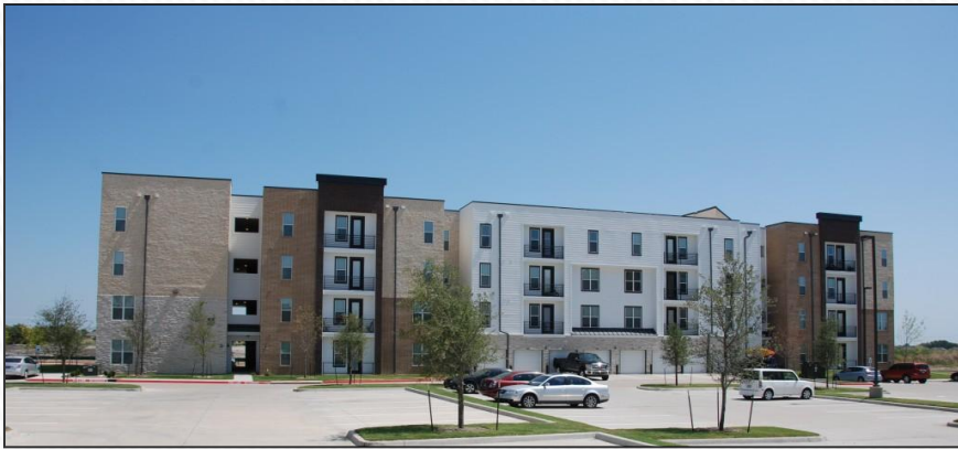
Millennium McKinney/Post Oaks Dallas HA – 13 Voucher Units
