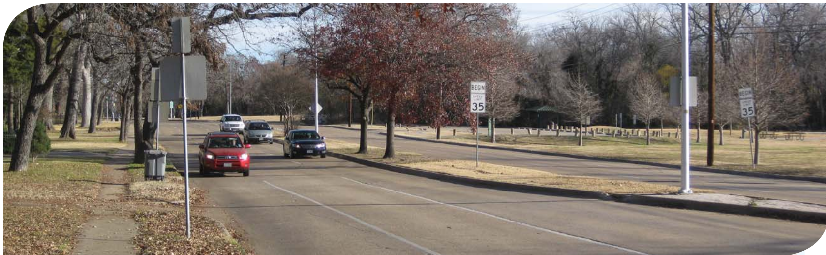
East Lake Highlands Drive at North Buckner Boulevard—six-lane divided thoroughfare
