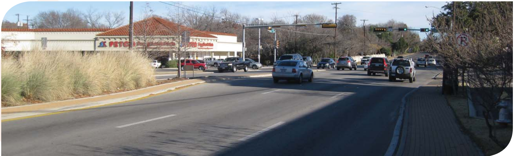
Garland Road at Buckner Boulevard—six-lane divided thoroughfare with bus stops, sidewalk, crosswalks, and planting zone
