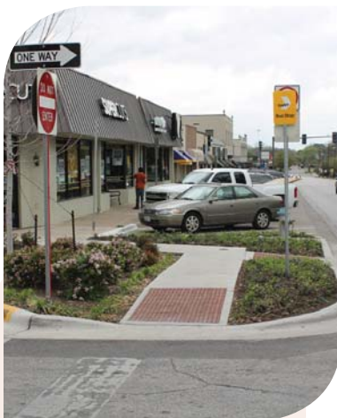
Near-side bus bulb on Hillcrest
