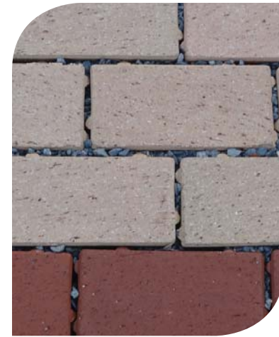
Pedestrian crosswalk with special pavers
