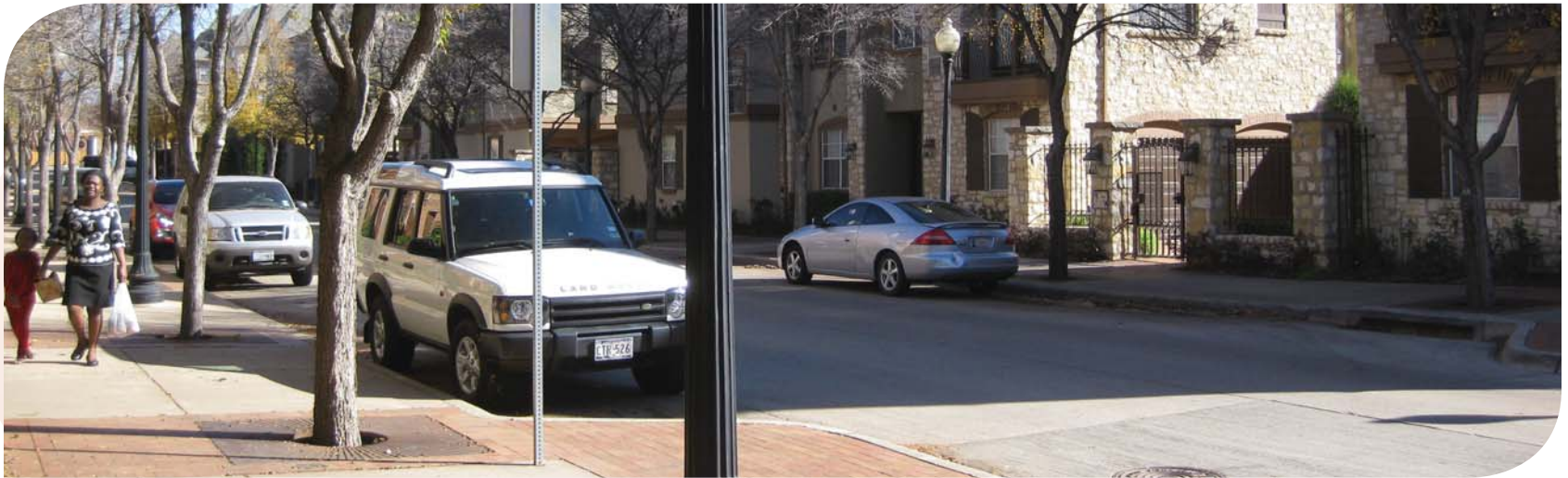
State Street at Ellis Street—two-lane street with on-street parking, buffer, and sidewalk
