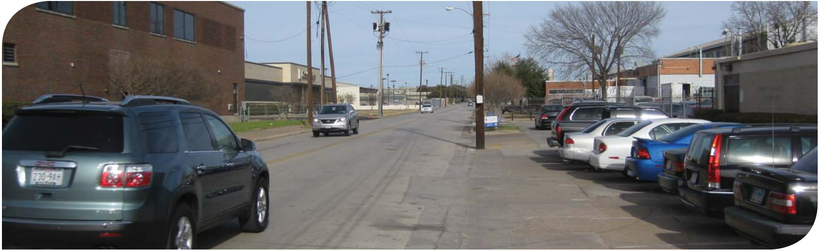
Manor Way at Cedar Springs Road—two-lane street
