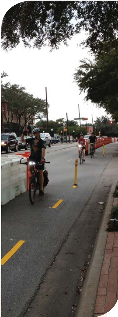
Knox Street demonstration project installed and monitored the operation of a two-way cycle track.
