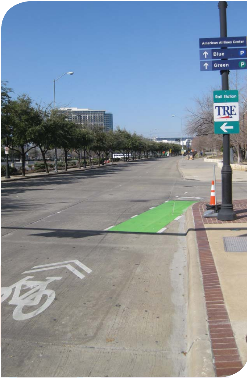
Bicycle and transit facilities—when integrated—typically exist in a symbiotic relationship. That is, each mode generates additional usage for the other mode.
