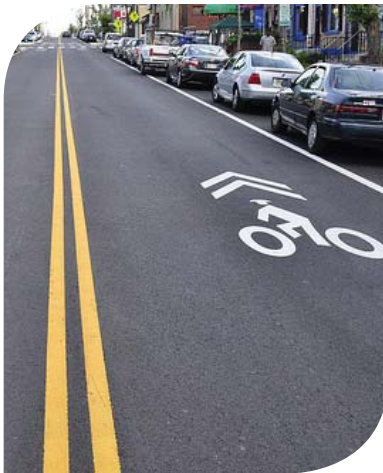
Shared lane marking
