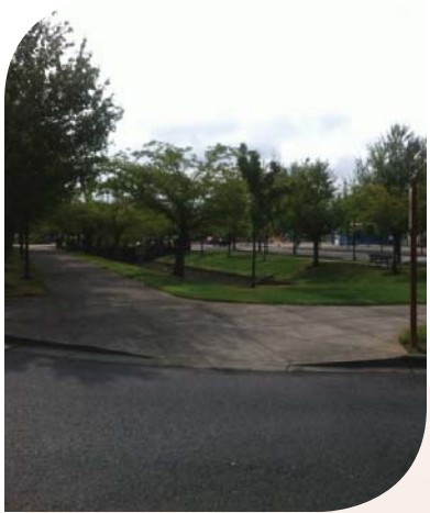
Stormwater can be retained and filtered in the medians of boulevards
