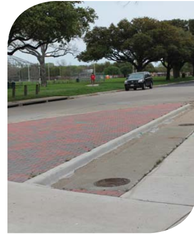
Diverter detail showing drainage design
