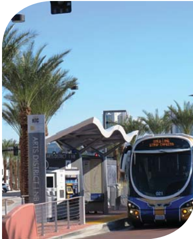
Bus Rapid Transit (BRT) stops typically feature an array of passenger amenities.
