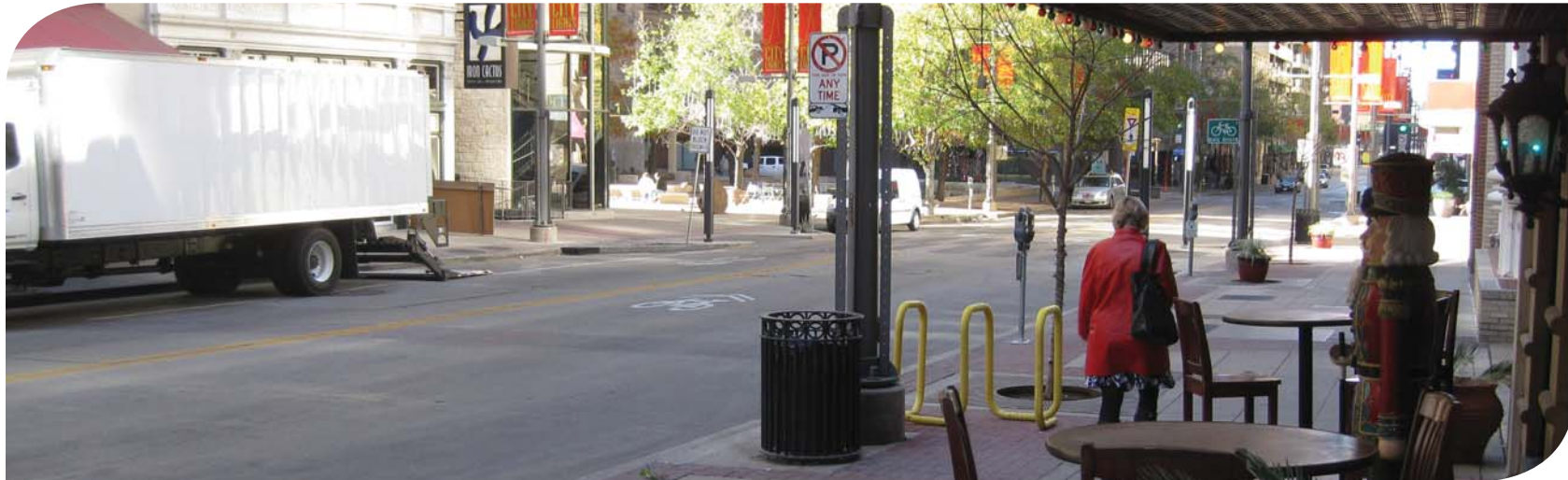
Main Street at Akard Street—two-lane thoroughfare with on-street parking
