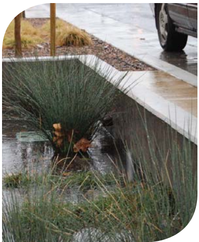
Permeable brick pavers
