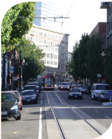
Safe and accessible designs for all modes of transportation must guide intersection design.
