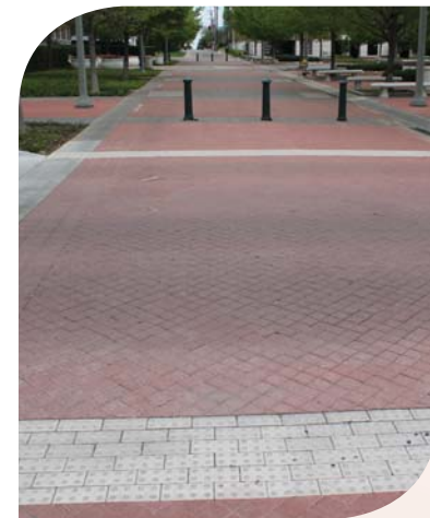
Pedestrian crosswalk with special pavers
