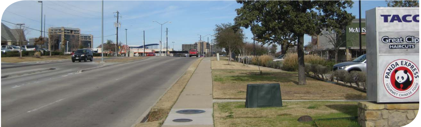
Montfort Drive at Belt Line Road—four-lane divided with sidewalk and buffer
