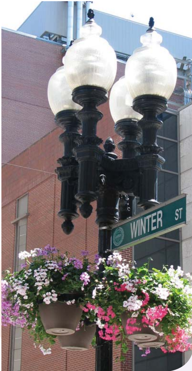
Minimum vertical clearances must be adhered to in cases of planter installations.
