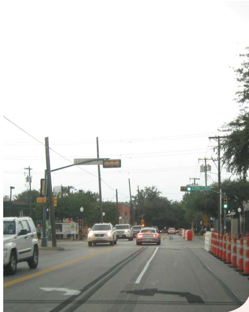
The Knox Street demonstration used blackout tape to temporarily cover up existing pavement markings.
