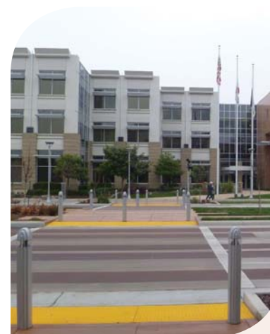
Major thoroughfare curb ramps
