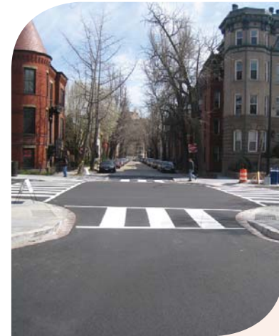
Clearly marked crosswalks and bulbouts increase pedestrian safety.
