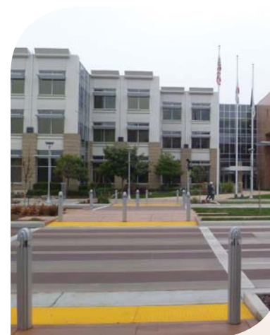
Pedestrian crosswalk with special pavers
