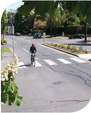
New crossing median island
