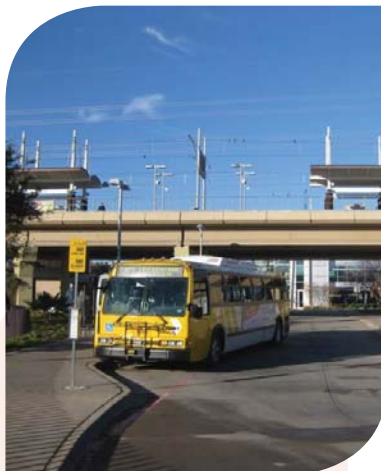
Bus bays allow a bus to pull out of travel lanes; typically at park-and-ride facilities.
