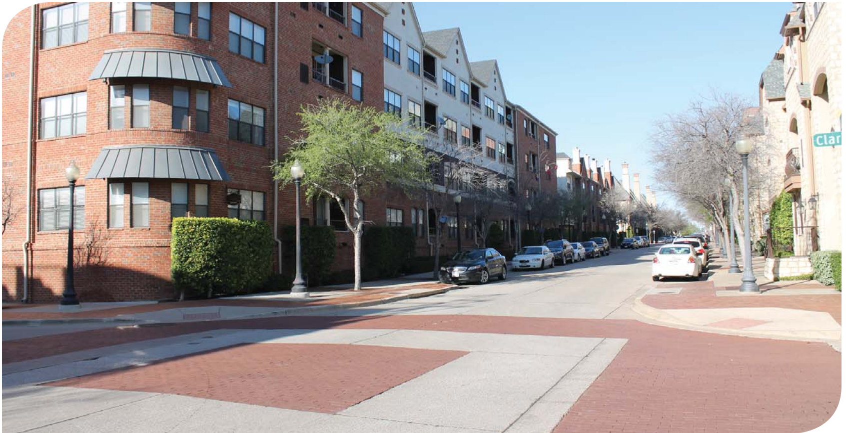
Textured paving materials notify drivers of the possible presence of pedestrians.
