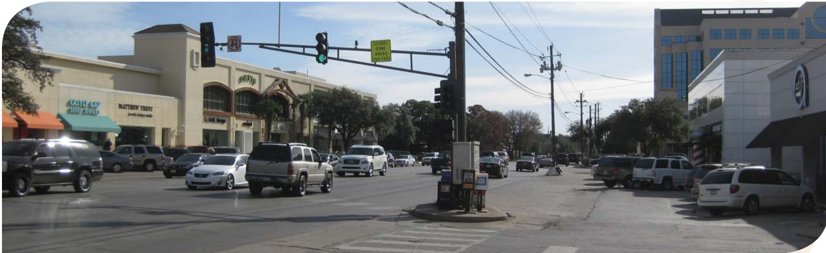
Preston Road at Weldon Howell Parkway—four- and five-lane thoroughfare with sidewalk, buffer, and off-street parking adjacent to commercial in a slip street format
