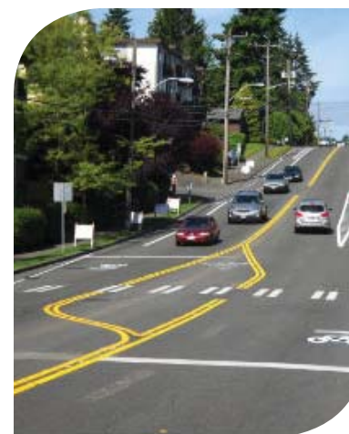
Bike lane and buffer transition at intersections
