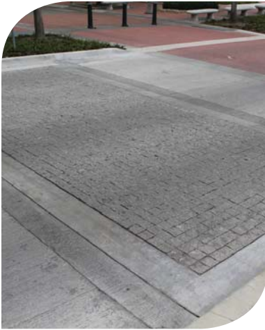
Textured crosswalk pavement
