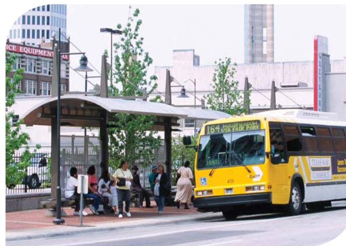
Stops should provide a clear sight line between operators and passengers.
