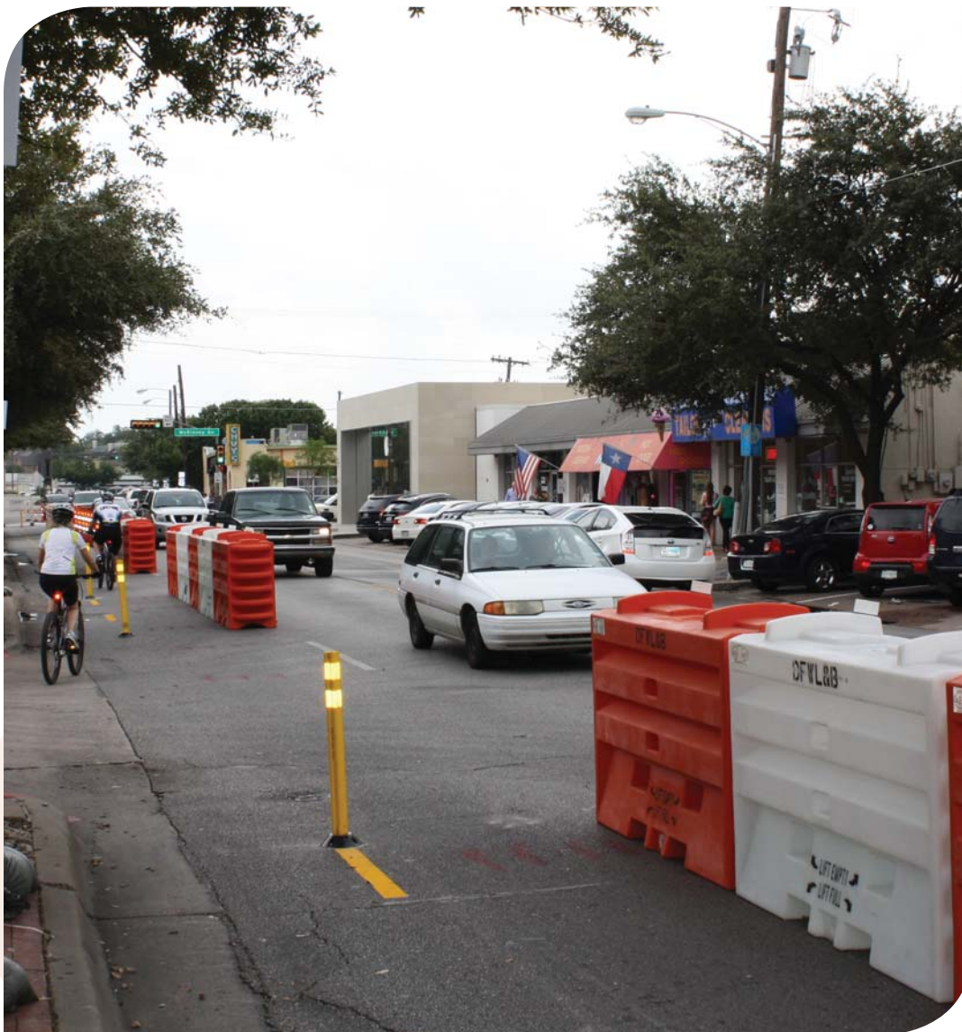
The Knox Street demonstration tested the installation of an eight-foot cycle track.
