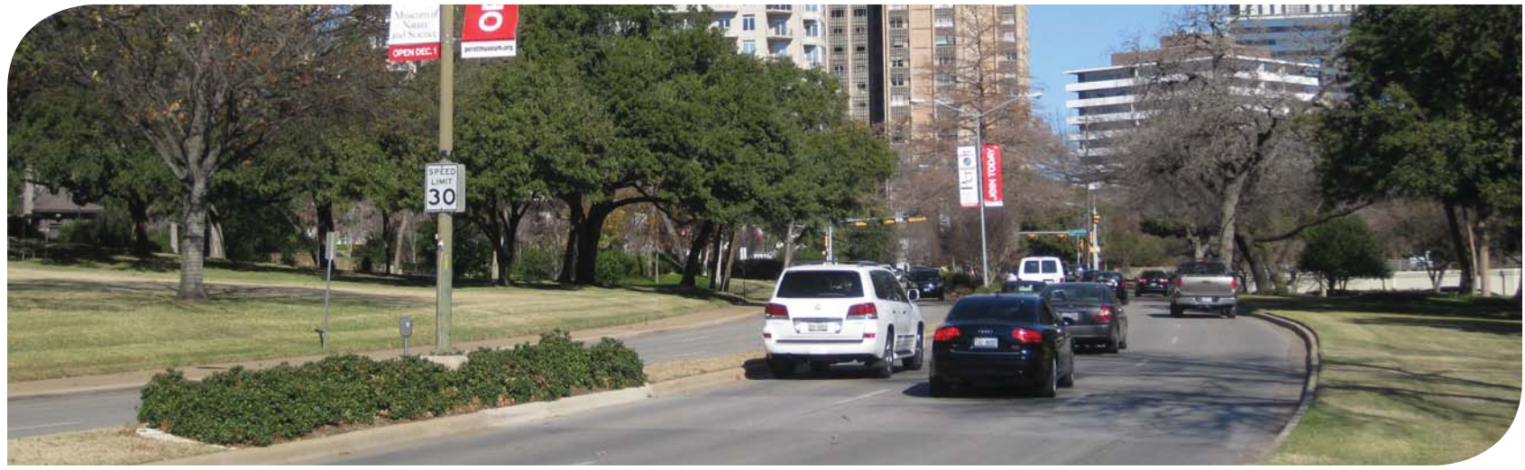
Turtle Creek Boulevard at Hall Street—six-lane divided thoroughfare
