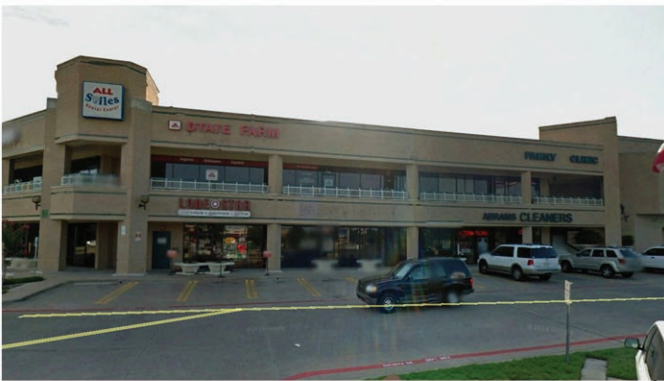
VIEW 2 -- EXISTING BUILDING IMAGE
