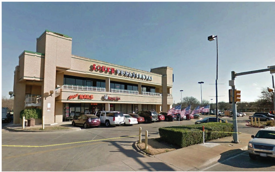
VIEW 1 -- EXISTING BUILDING IMAGE
