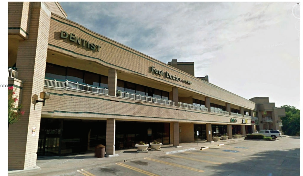
VIEW 5 -- EXISTING BUILDING IMAGE
