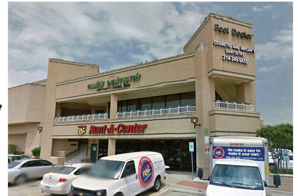
VIEW 4 -- EXISTING BUILDING IMAGE
