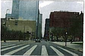
Figure 17: Main Street between Houston & Market, looking east
