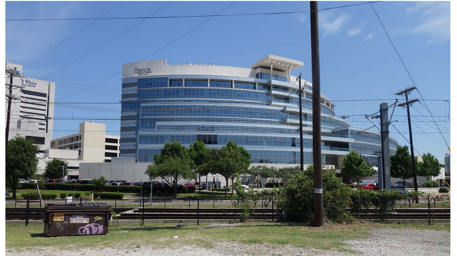
12. BAYLOR CANCER CENTER LOOKING NORTH FROM TRUNK AVENUE
