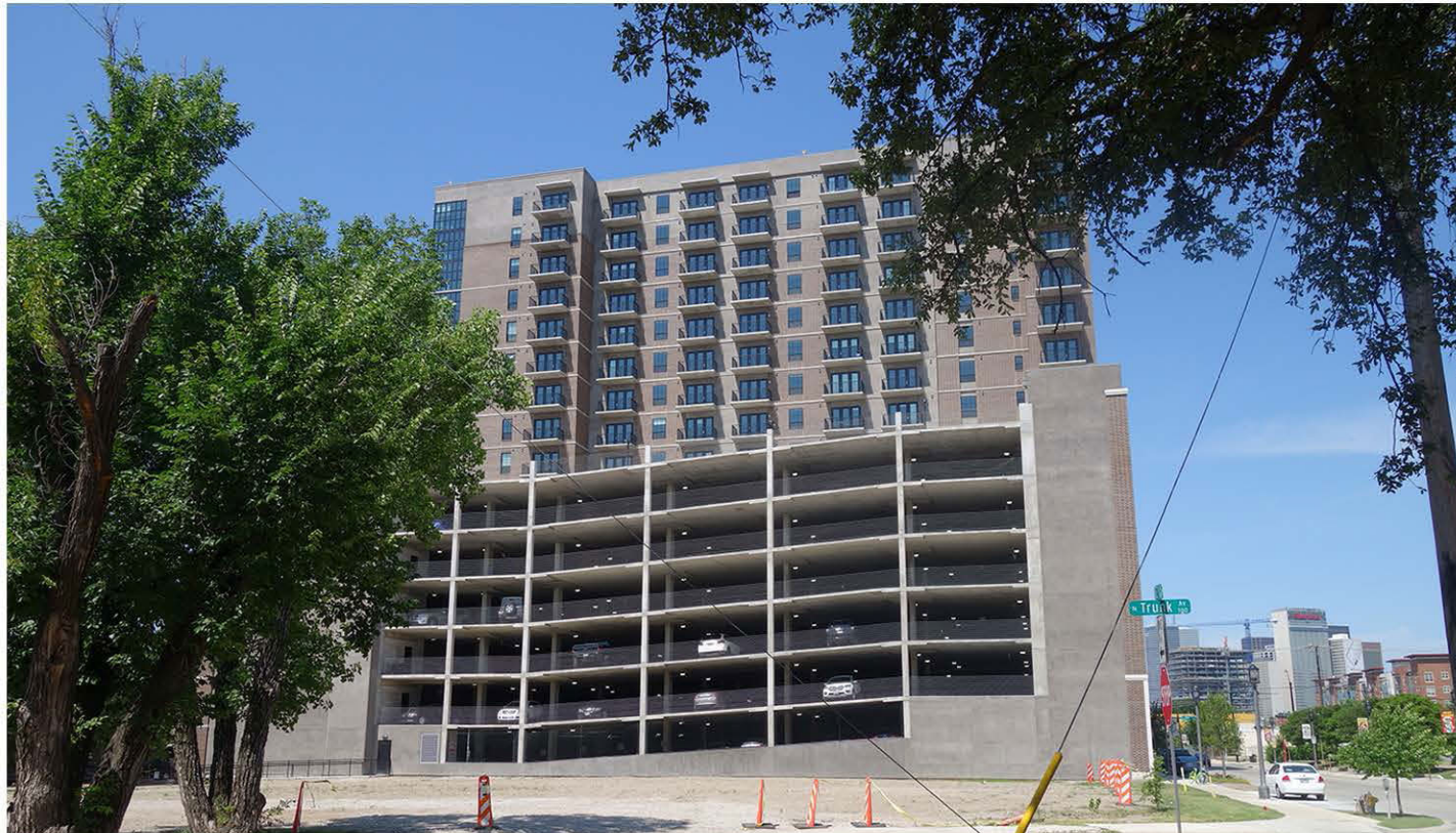
13. CASE BUILDING LOOKING WEST FROM TRUNK AVENUE AND ELM STREET
