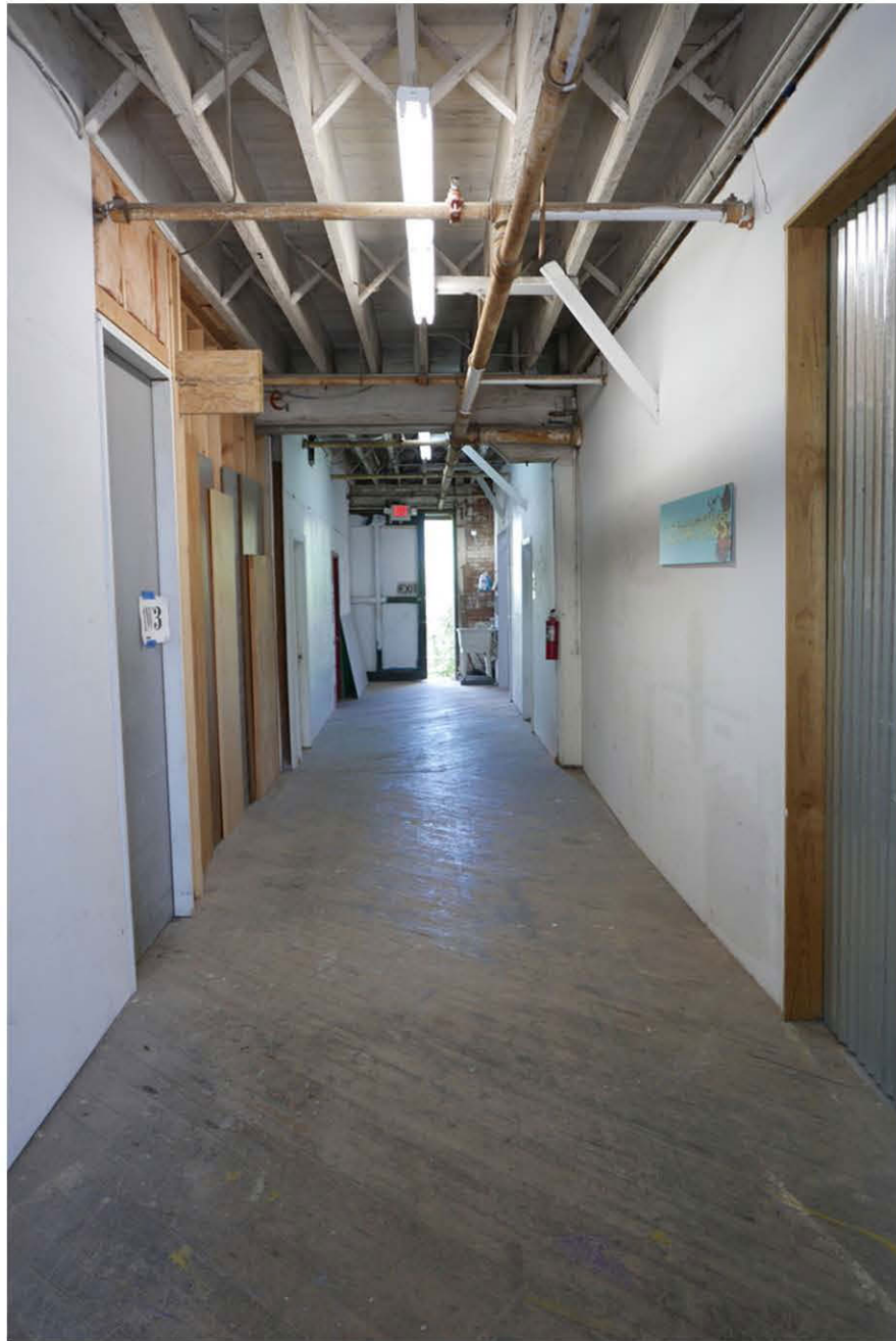
GROUND FLOOR LOADING AREA
