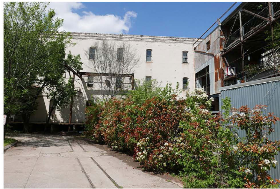
CONTINENTAL GIN BUILDING VIEW FROM THE SOUTH
