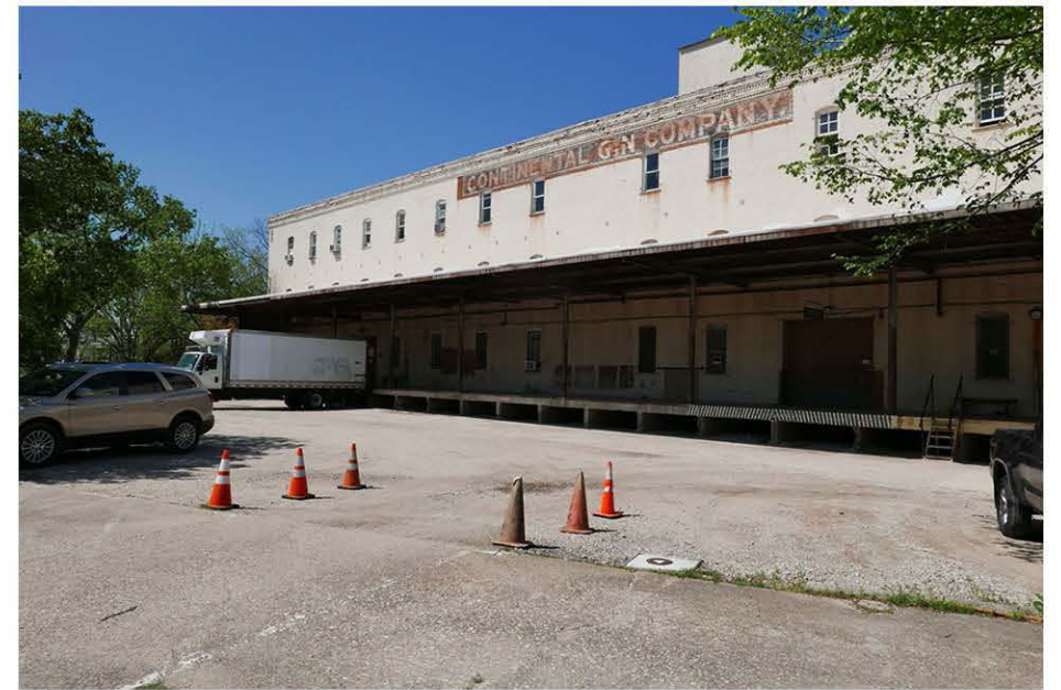
CONTINENTAL GIN BUILDING VIEW FROM THE SOUTH
