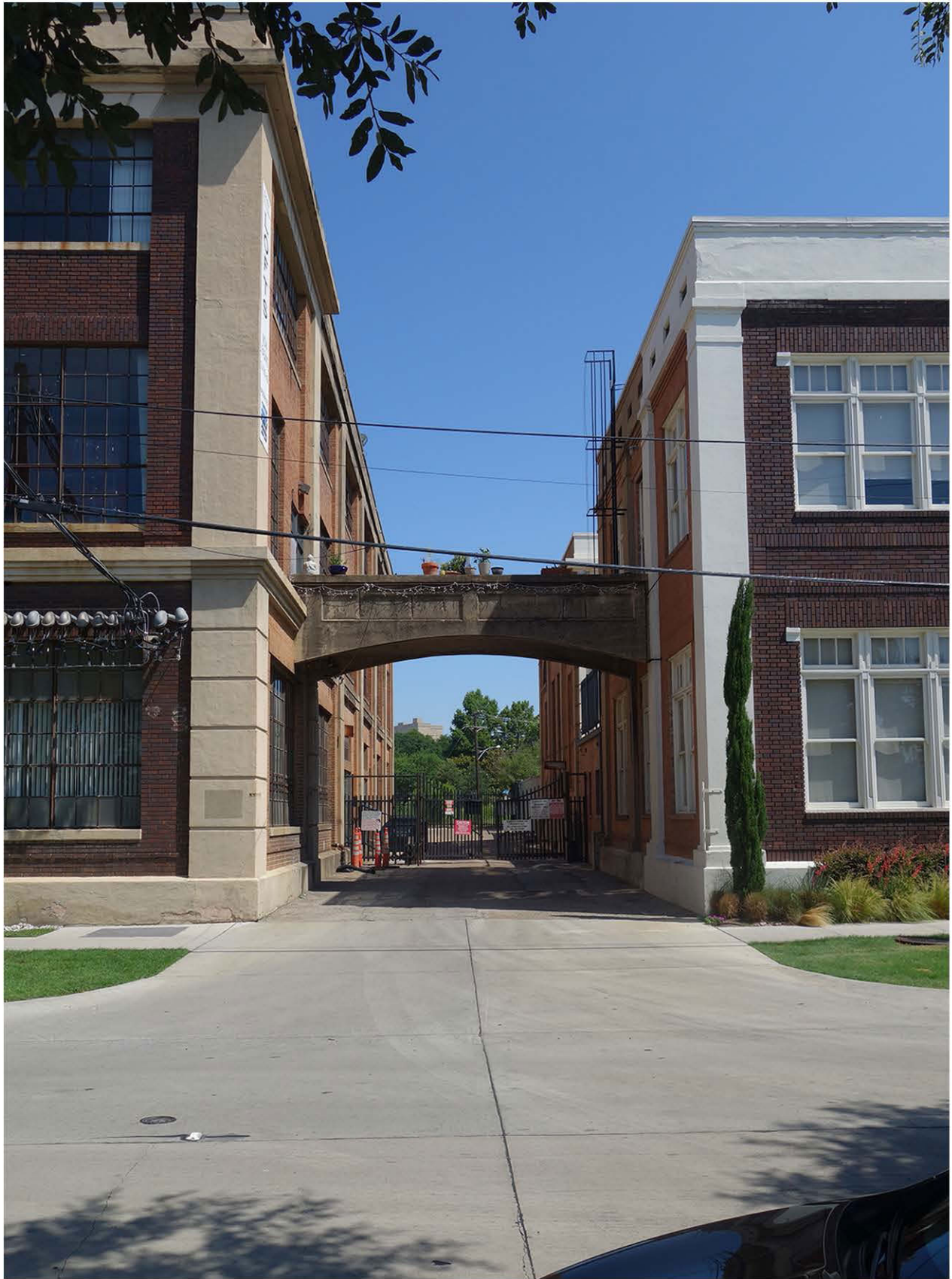
4. CONNECTING BRIDGE OVER DRIVE BETWEEN 3311 ELM AND 3333 ELM
