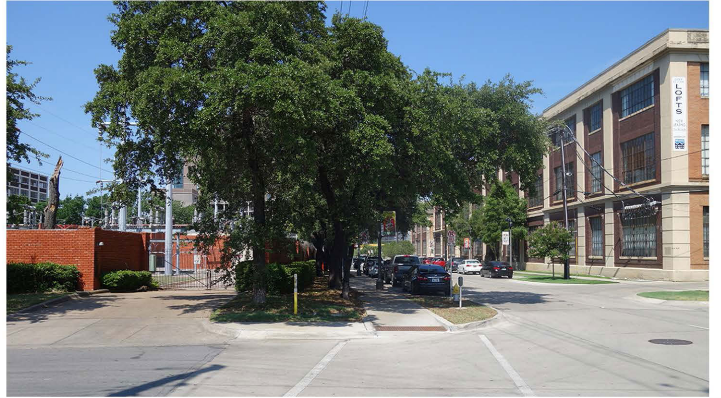
2. 3311 ELM AND POWER STATION LOOKING WEST FROM ELM STREET
