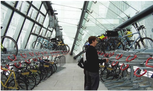
The Union Station METRO in Washington DC has a large, protected bike storage facility
