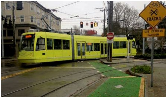
This bike lane crosses the light rail track at a near 90° angle, protecting cyclists from falls
