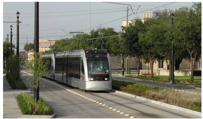
The light rail in Houston has large truncated domes protecting the transit lane from the travel lane
