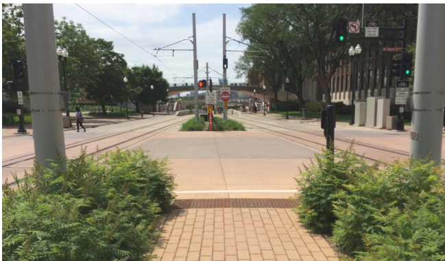
This light-rail platform leads to a large crosswalk that is paved with a different, distinguishable material
