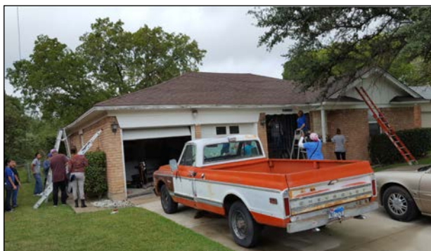
Volunteers repair a home in Pemberton Hill
