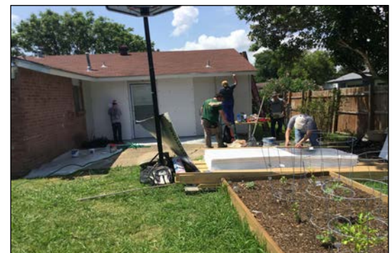
World Changers volunteers repair a home in Pemberton Hill
