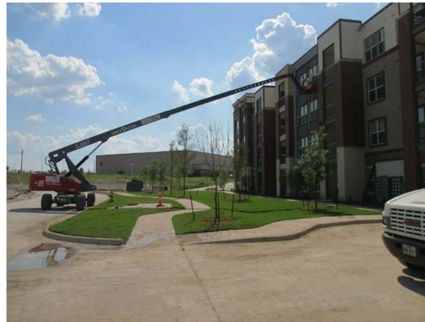
02. LOOKING FROM NORTHWEST
