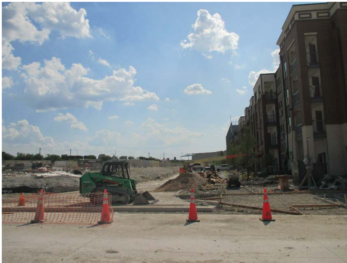
09. LOOKING FROM NORTHWEST
