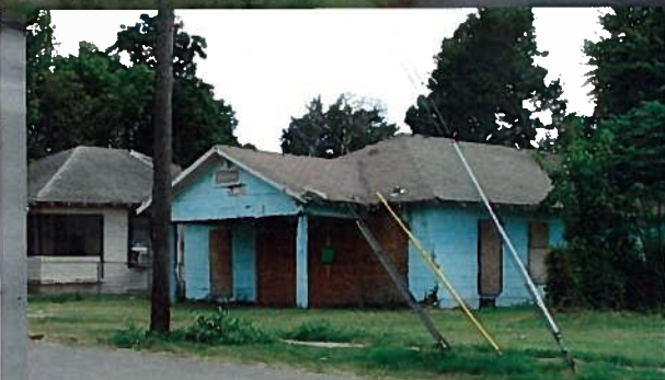
Typical abandoned house along the corridor
