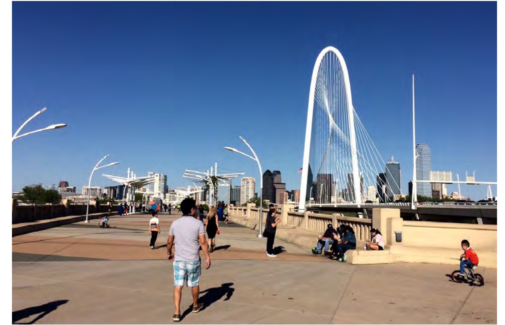
The Ronald Kirk Bridge crosses over the Trinity River, connecting the Design District to West Dallas.
