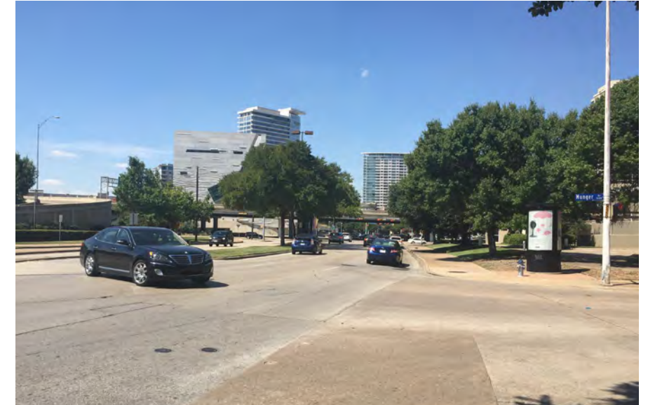
The Griffin/ Field intersection is complicated, making it unsafe for pedestrians and drivers.
