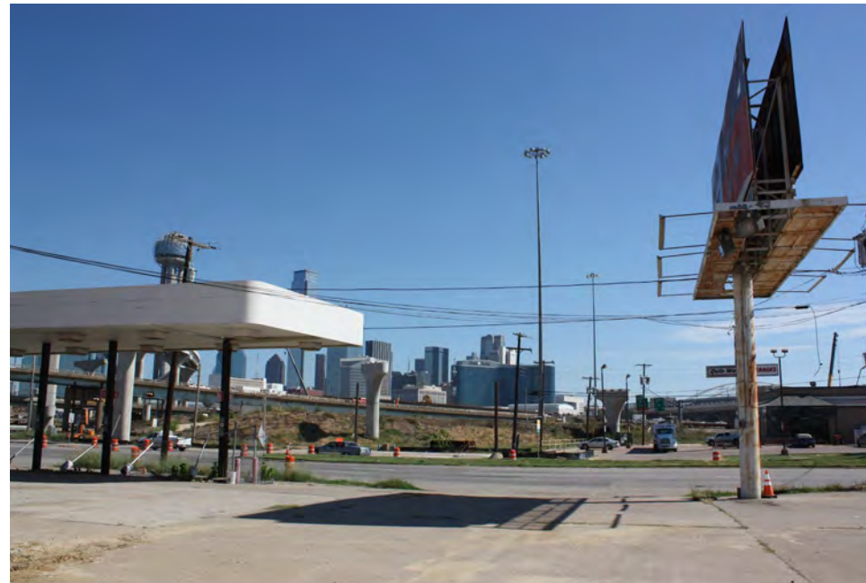
Although Downtown is roughly a half-mile away, Riverfront is isolated by the TxDOT Horseshoe Project and other large infrastructure.
