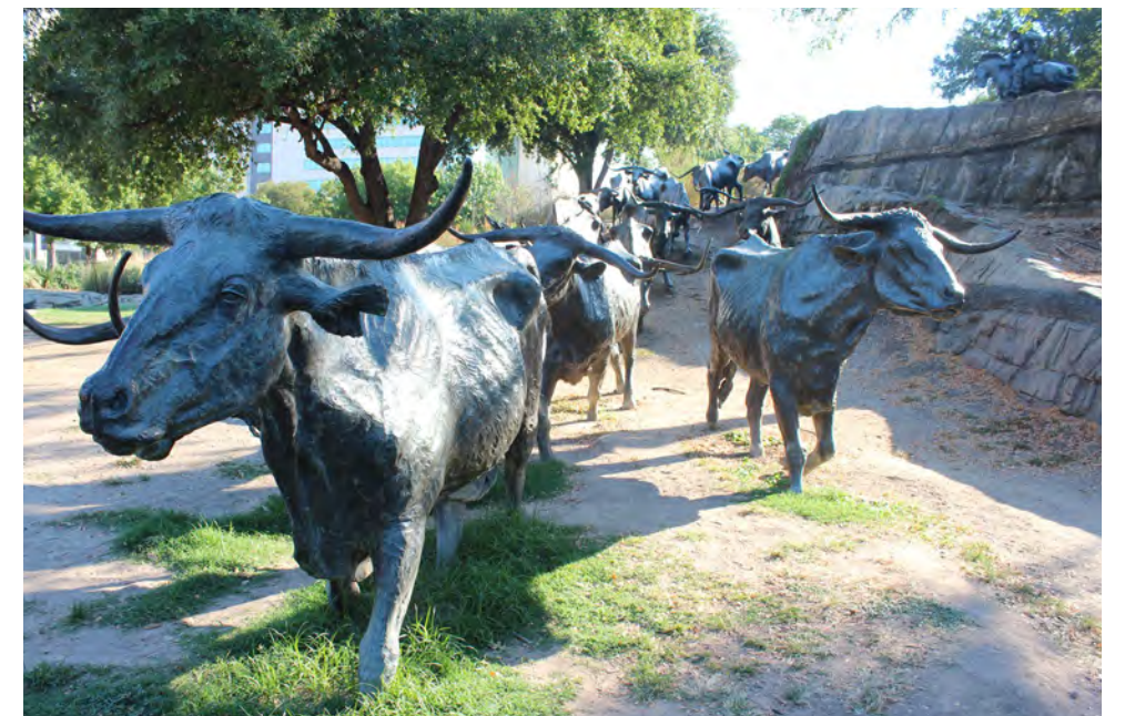
Due to heavy tourist traffic through Pioneer Plaza in the Civic Center, the paths around the iconic cattle drive sculptures and cemetery are eroded and need repair.
