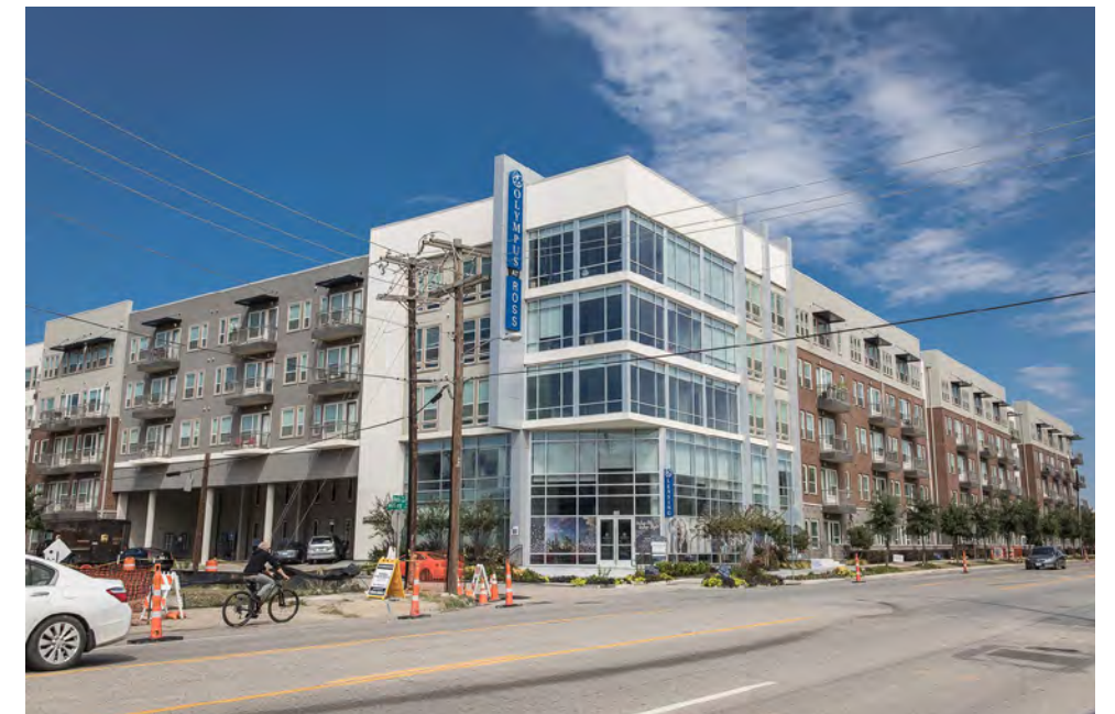
Numerous new multifamily developments have been built along Ross Avenue and Live Oak Street within the district.
