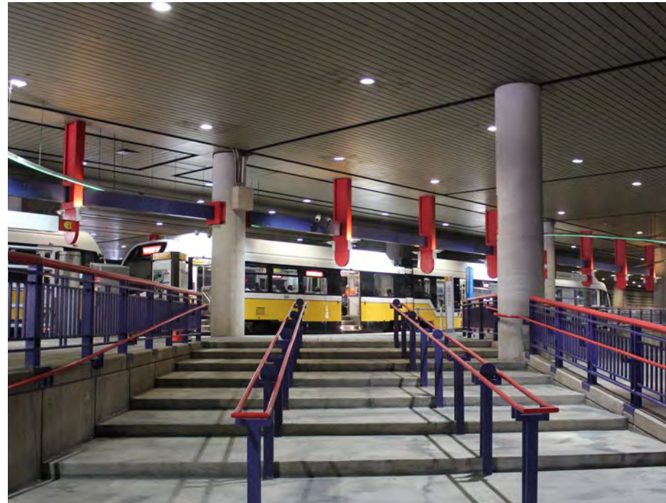
The underside of the Kay Bailey Hutchison Convention Center provides a great opportunity for creating an activated space that connects Downtown to the Cedars.
