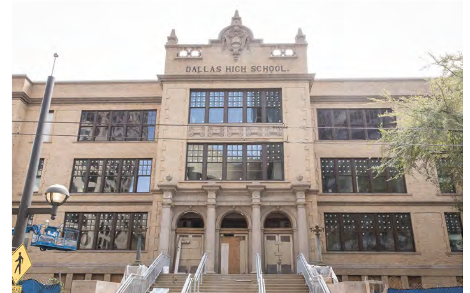
The renovation of Old Dallas High School preserves an outstanding historic building in the area and will provide a new anchor adjacent to the park.
