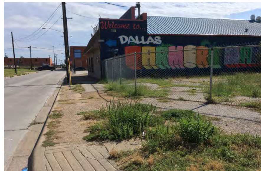
Poor sidewalk conditions exist throughout the area, making access to nearby amenities such as the Dallas Farmers Market difficult.
