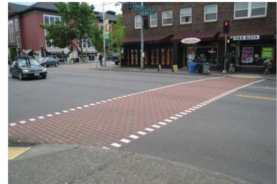
Example of a marked crosswalk
