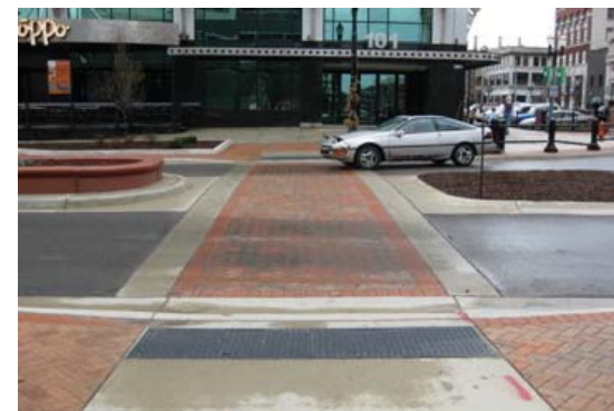
Example of a marked crosswalk
