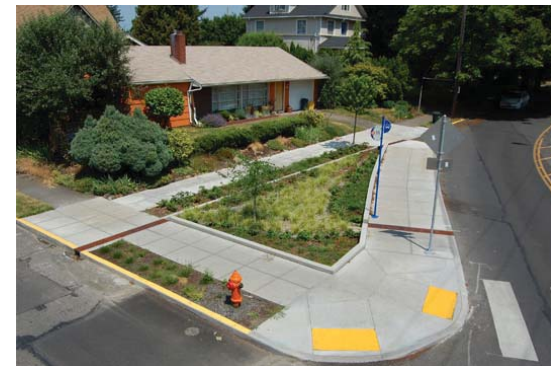
Street park at street corner
