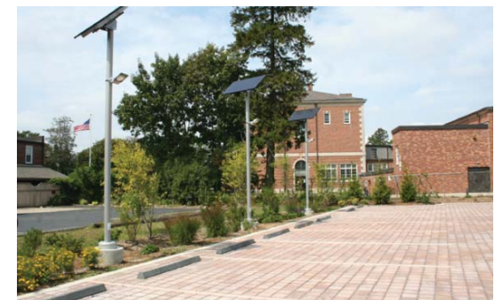
Examples of surface lots that enhance the public realm through their location, limited size, surface treatment, and landscaping
