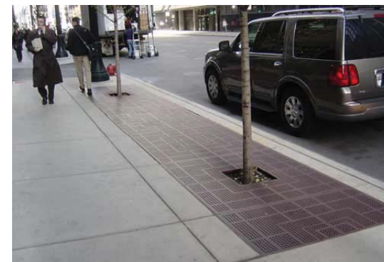
Use of tree wells on a heavily traveled city sidewalk.
