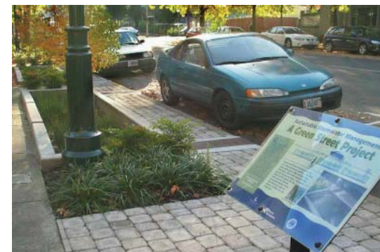
A sustainable stormwater management system incorporated into the design of a street
