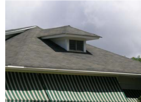
A hipped dormer has a roof with flat surfaces that slope upward at the front of the dormer as well as on both sides.
