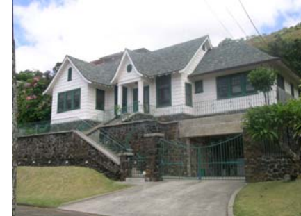
Bellcast eaves or flared eaves are the part of the roof that has a gradually diminishing slope and projects beyond the face of an exterior wall, flaring upward near its lower end. Flemish in origin.
