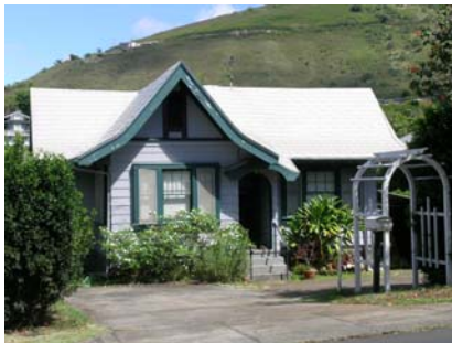
Bellcast eaves or flared eaves are the part of the roof that has a gradually diminishing slope and projects beyond the face of an exterior wall, flaring upward near its lower end. Flemish in origin.
