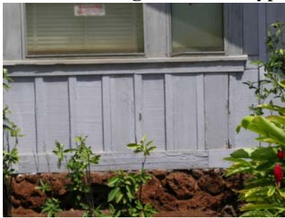
Board-and-batten is lapped siding.
