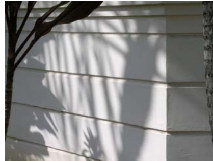
Drop siding has a simple channel
