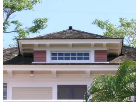
A hipped dormer has a roof with flat surfaces that slope upward at the front of the dormer as well as on both sides.
