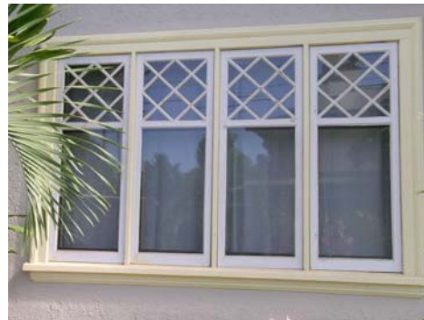
If sash windows pivot about a vertical axis, they are casement windows.
