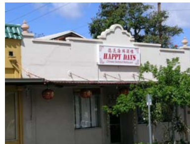
Curvilinear parapeted gable
