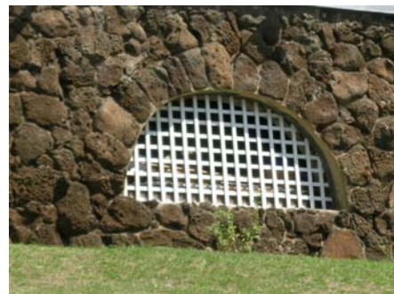
Lattice foundation vent
