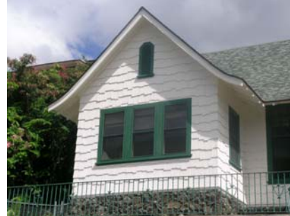
Bellcast eaves or flared eaves are the part of the roof that has a gradually diminishing slope and projects beyond the face of an exterior wall, flaring upward near its lower end. Flemish in origin.
