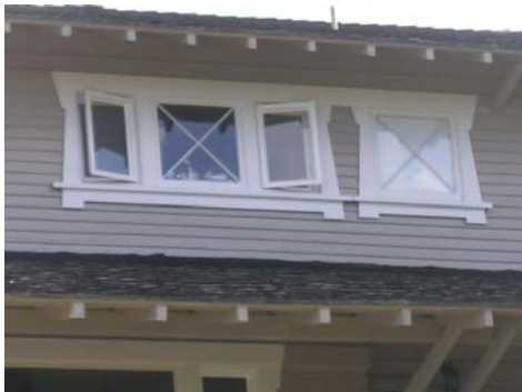
If sash windows pivot about a vertical axis, they are casement windows.
