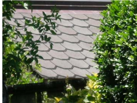
Slate fish-scale shingles
