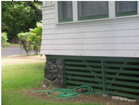
Wood-slat foundation vent
