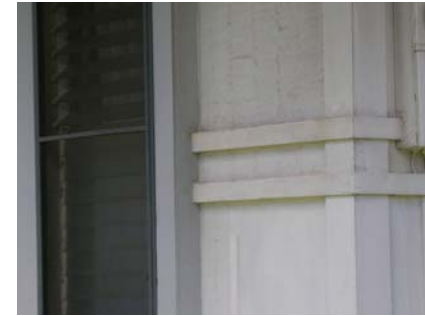
Tongue-and-groove (T & G) boards
