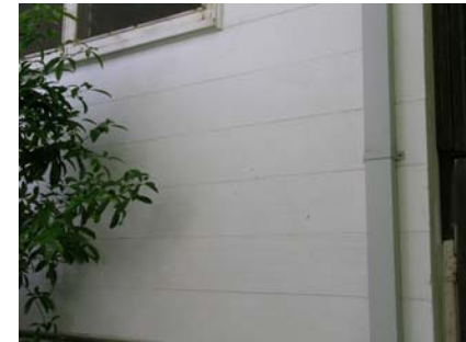
Tongue-and-groove (T&G) boards
