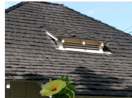
Wood slat attic vent
