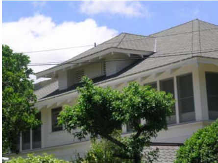
A hipped dormer has a roof with flat surfaces that slope upward at the front of the dormer as well as on both sides.
