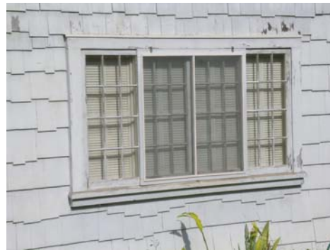
A sash window that moves in a horizontal plane is a sliding sash window.
