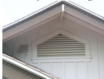
Louvered gable vent
