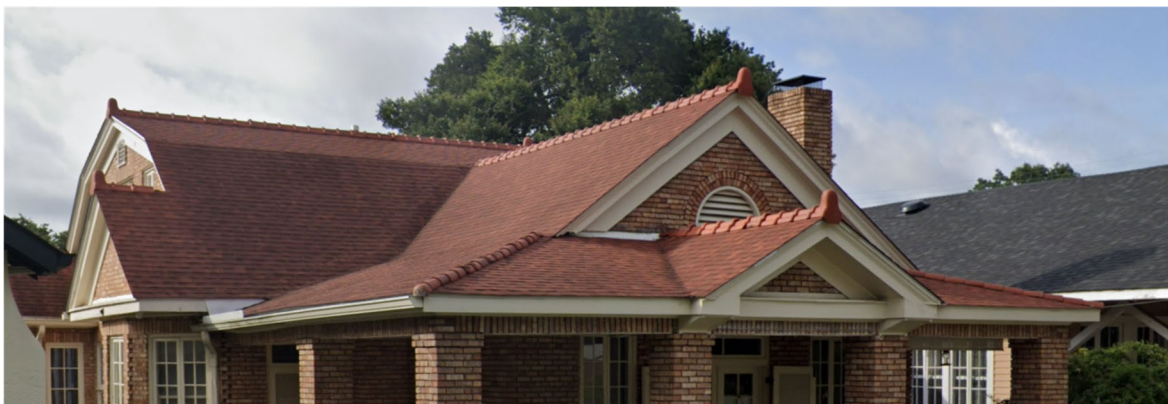
Example: Composition shingles in a color palette of original Spanish tile roofs with terra cotta hips, ridge caps, and rake tiles applied to mimic original tile roofs.
