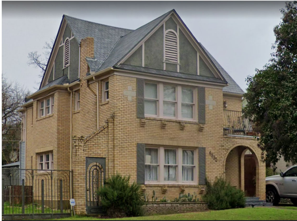
1-over-1 ; Ganged windows separated by wood mullion
