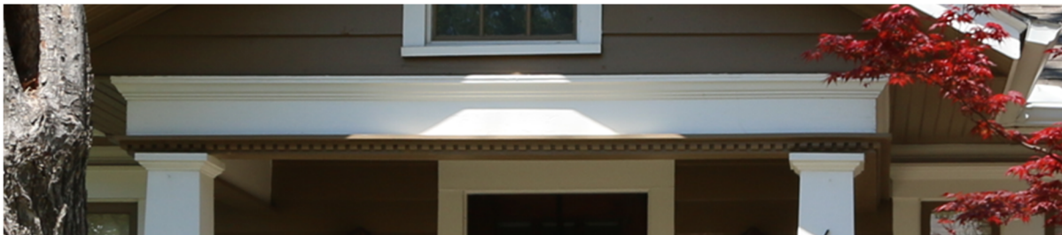
Examples: Minimum 8-inch header beam.
