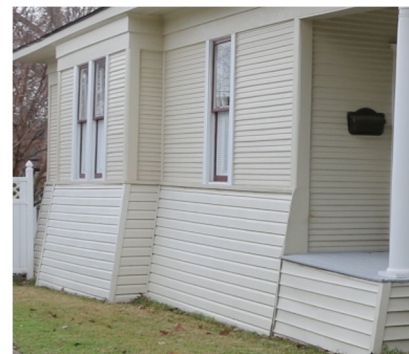
Example: Battered or sloped skirting.
