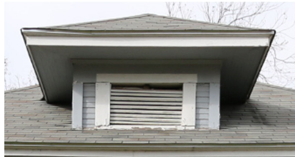
Example: Hipped dormer with louvered vent.
