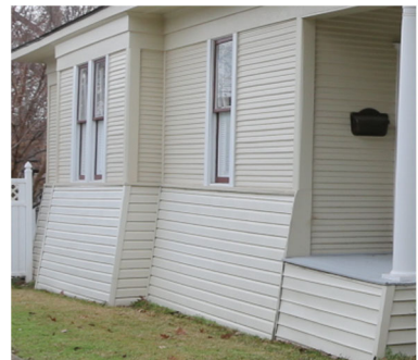
Example: Battered or sloped skirting.
