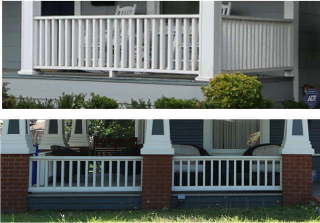
Examples: Wood balustrade on the front porch.
