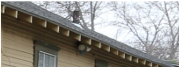
Examples: Exposed rafter tails
