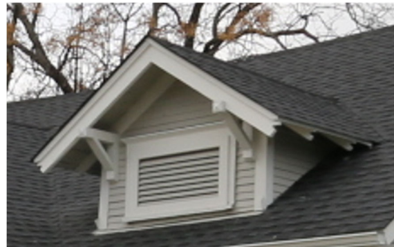
Example: Gabled dormer with louvred vent window.
