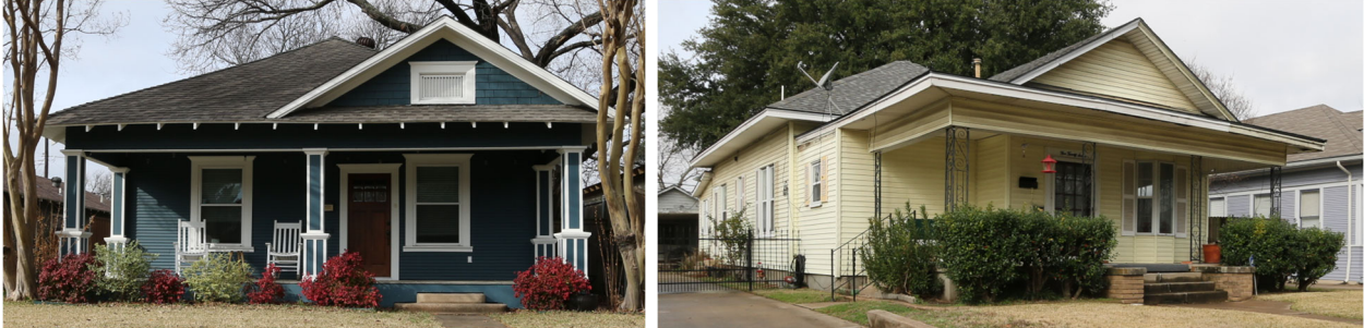
Examples: Recessed gable above the front porch.
