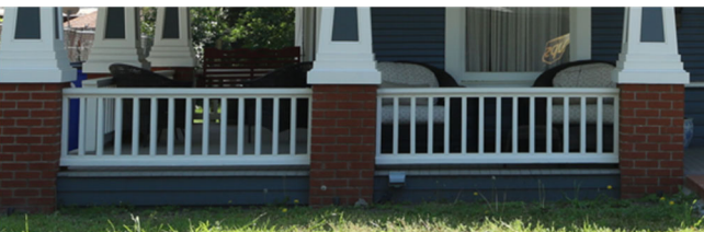
Examples: Wood balustrade on the front porch.
