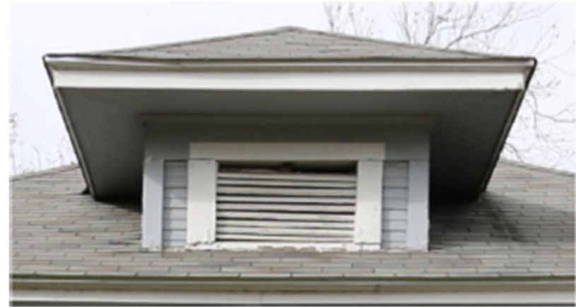
Example: Hipped dormer with louvred vent.
