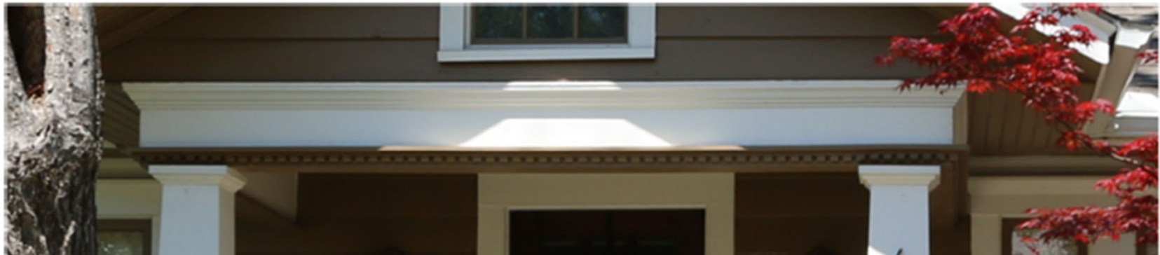
Examples: Minimum 8-inch header beam.
