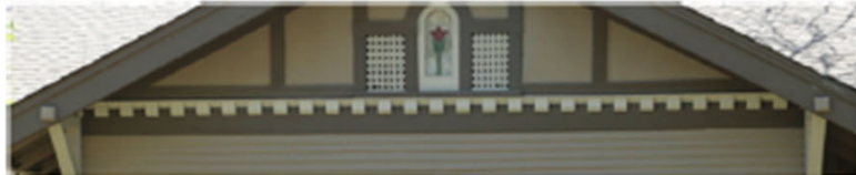
Examples: Dentil molding.
