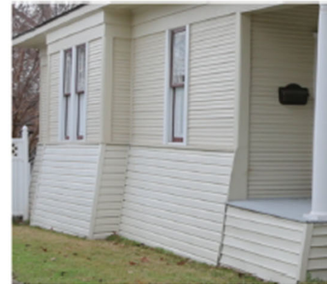
Example: Battered or sloped skirting.
