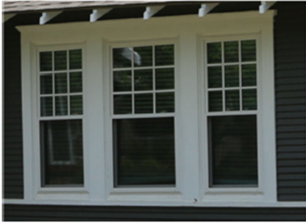
Example: Windows with divided light upper sash.
