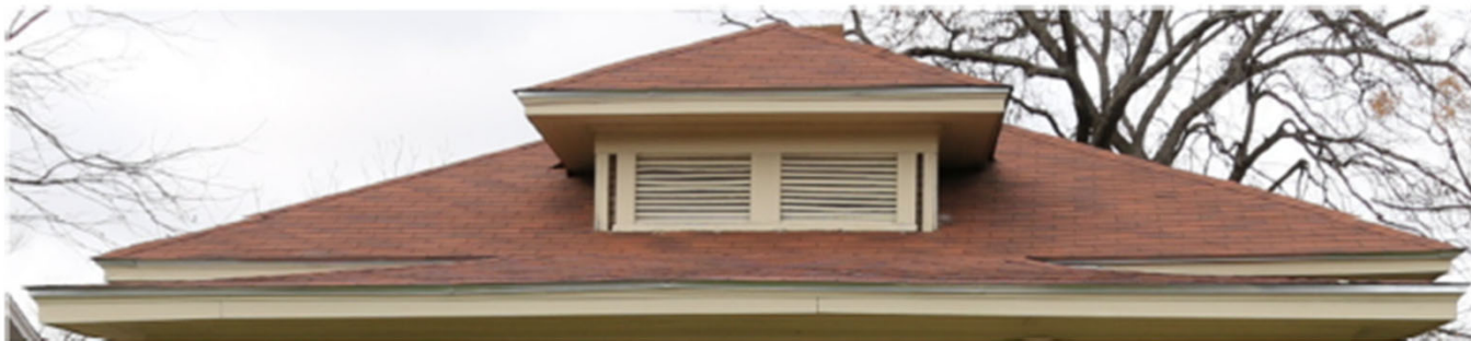
Examples: Centered, hipped dormer with louvered vent.
