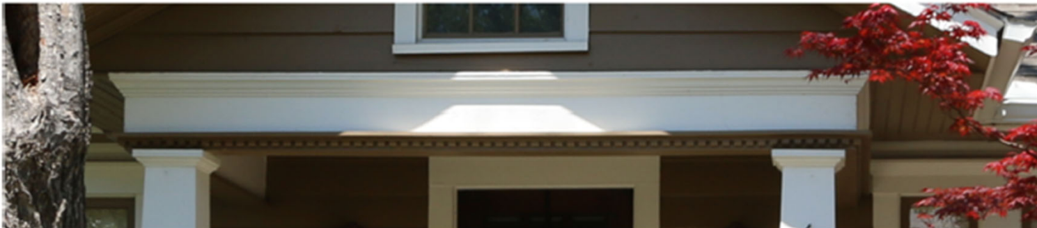
Examples: Minimum 8-inch header beam.
