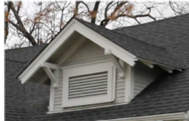
Example: Gabled dormer with louvred vent window.
