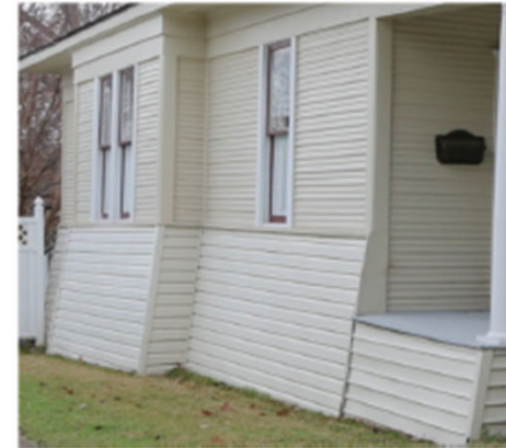
Example: Battered or sloped skirting.
