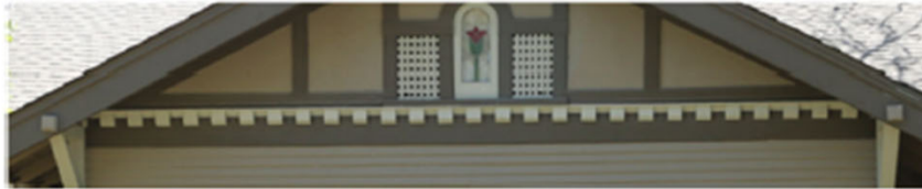
Examples: Dentil molding.
