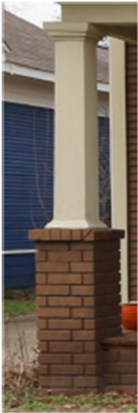
Examples: Typical column design and proportions for the Transitional Bungalow style.
