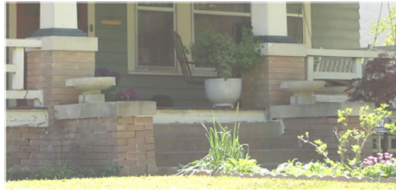
Example: Battered or sloped skirting.
