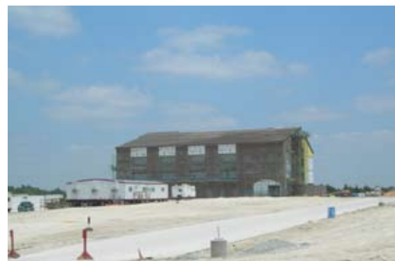
The new UNT Campus Master Plan provides for a build-out capacity of 25,000 students. The first building is under construction and scheduled to be opened in early 2007.
