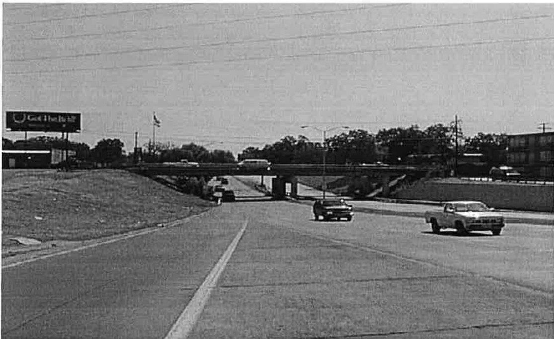
Existing Gateway Area at Denton Drive
