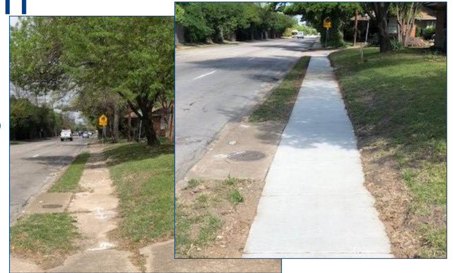
Example of Sidewalk program repairs
